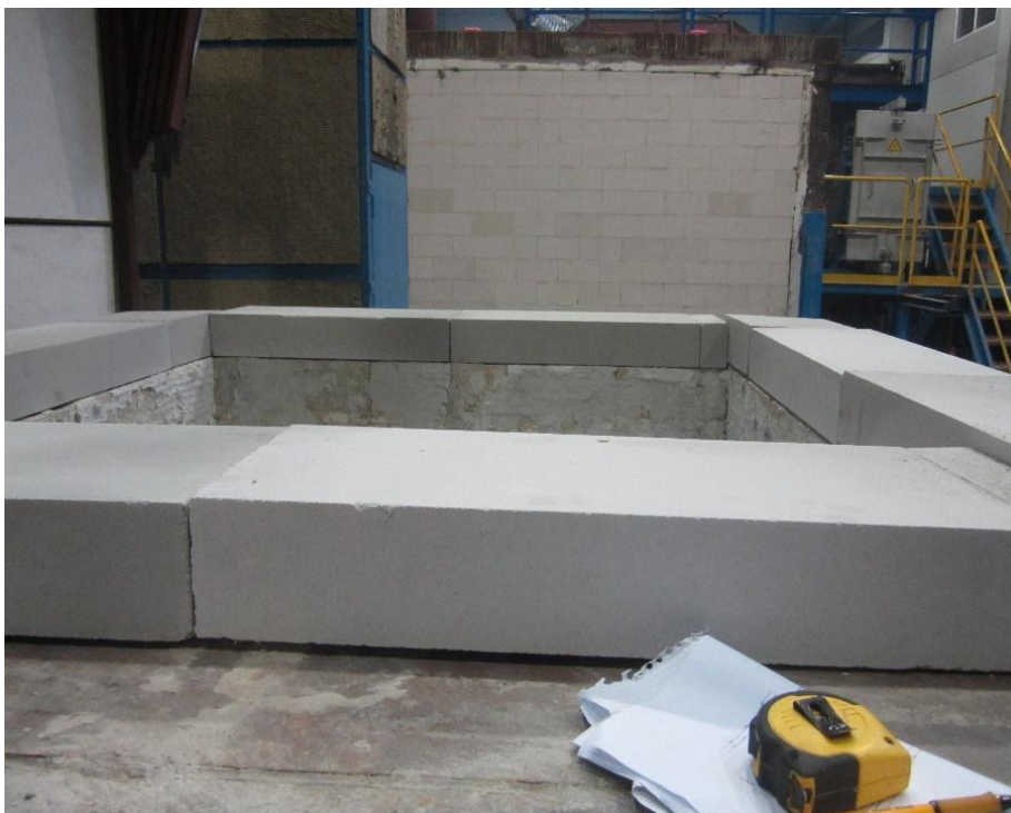
Figure 5.21 Top side furnace and AC blocks
