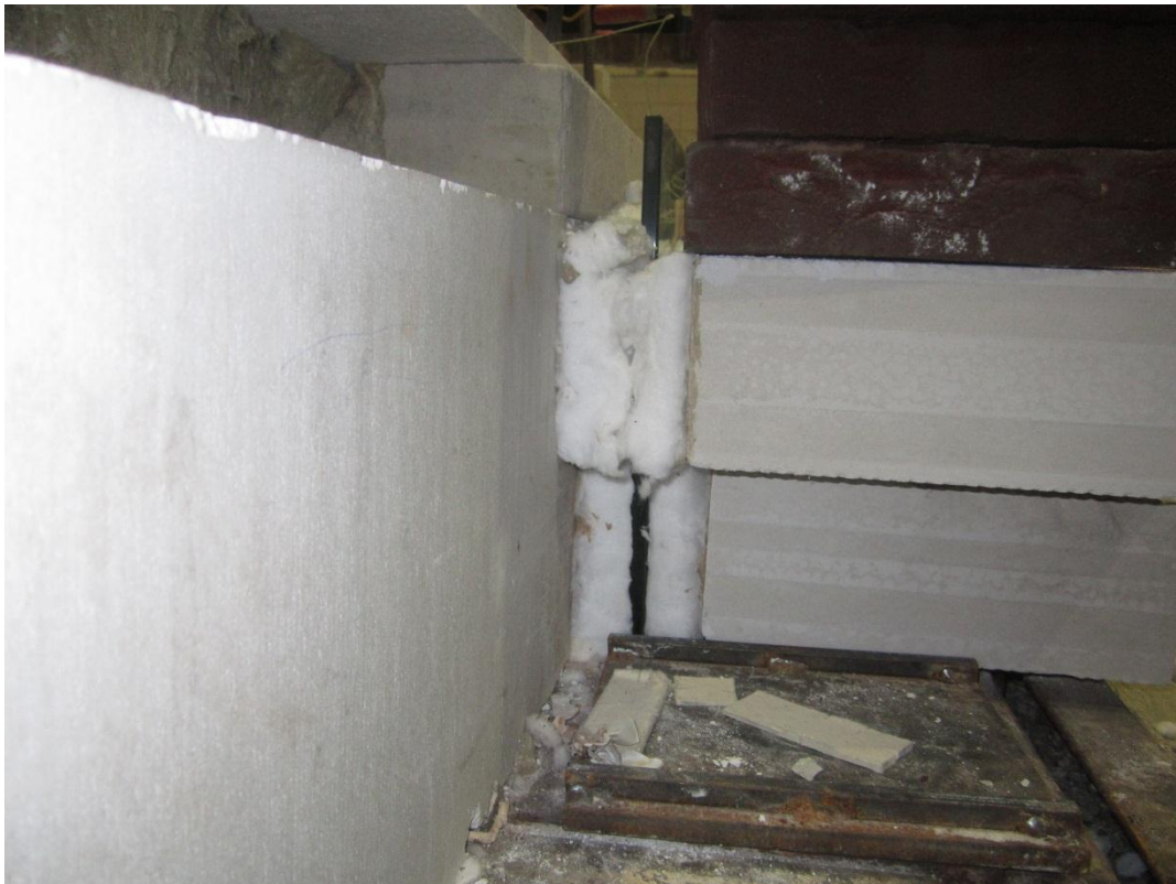
Figure 5.52 location of pane E between ACC beam and blocks
