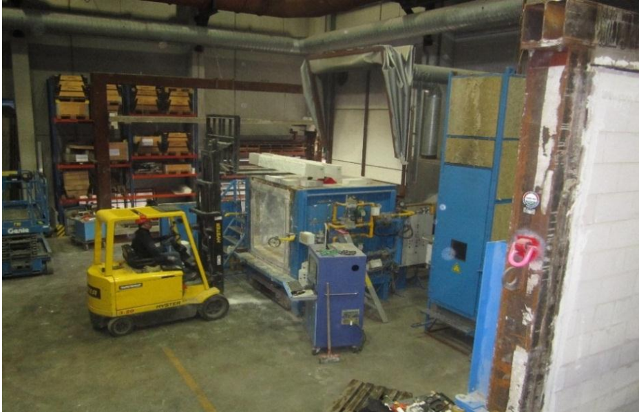
Figure 5.22 placing ACC beams at top side furnace
