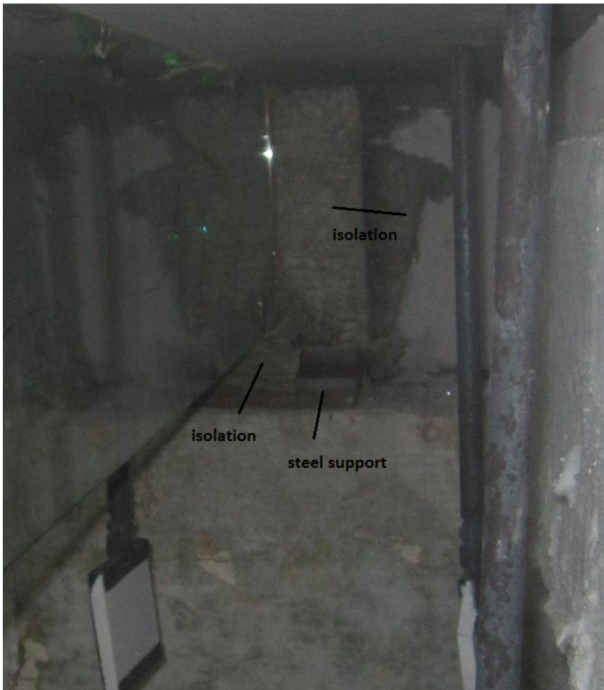
Figure 5.48 Isolation between glass and steel support
