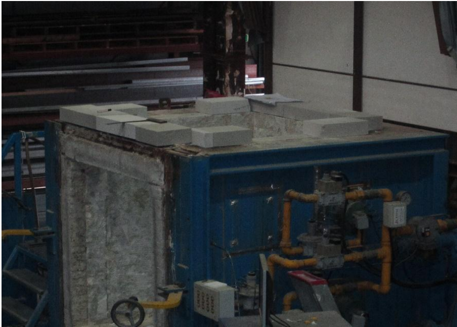
Figure 5.20 AC blocks placed on furnace edges
