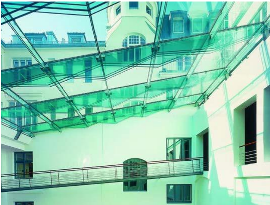
Figure 1.3 14 m span courtyard roof covering IHK Munich Engineering (F. P. Bos)
