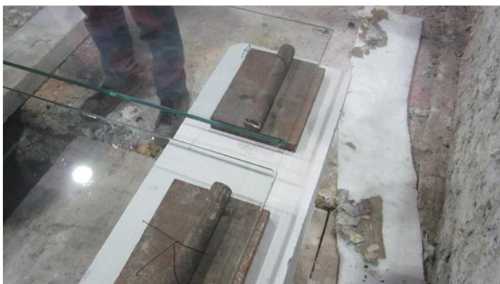
Figure 5.4 Glass panes and steel supports
