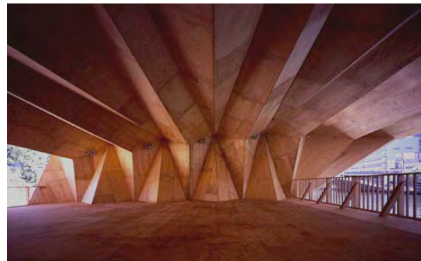
Ryuichi Ashizawa Architects. Folded structure at Aqua Metropolis Osaka Event Photo by RAA.
