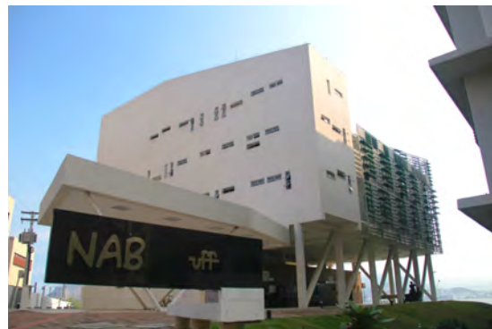
NAB - Niteroi: Office buildings analyzed. 2015.
