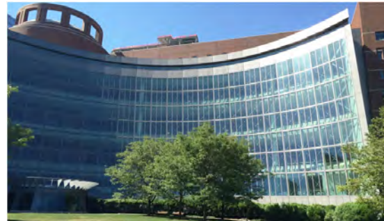
Glass façade with metal bracings at the John Joseph Moakley U.S. Courthouse in Boston, Massachusetts, United States
