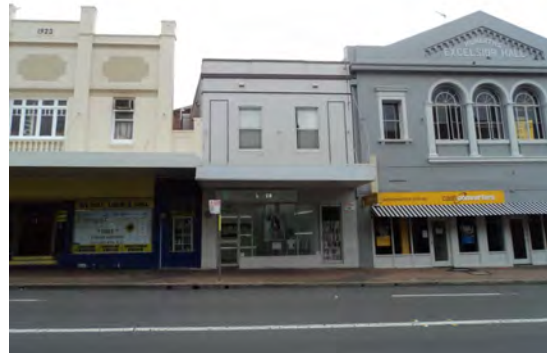
Fig. 2 Facades on Crown Street. Source: Google Maps. Accessed: 05-08-2016
