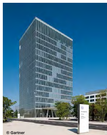
Figure 1: Roche Bau 5 with the first CCF in Basel .
