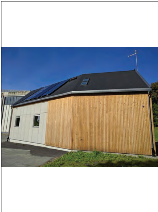
Fig. 1. The ZEB Test Cells Laboratory external view
