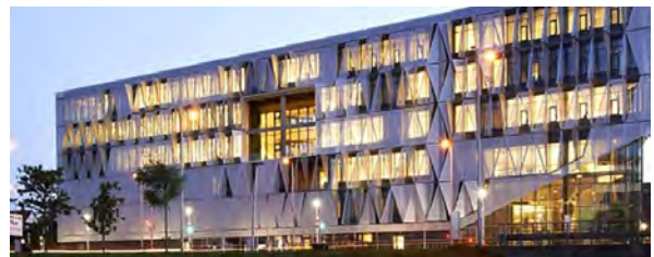
Kolding Campus, South of Denmark University, Denmark
