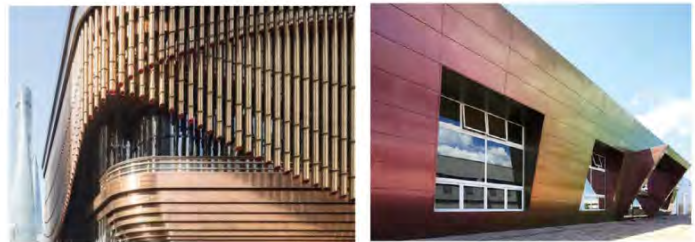
Material references: PVDF aluminium
