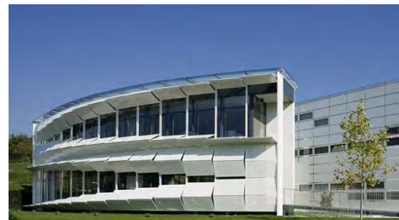
Dynamic facade (Kiefer Technic Showroom) Bad Gleichenberg, Autriche (source: https://www.architonic.com/fr )
