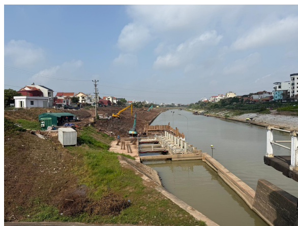
Figure 11.10: Construction of extra pump capacity at the Xuan Quan lock.
