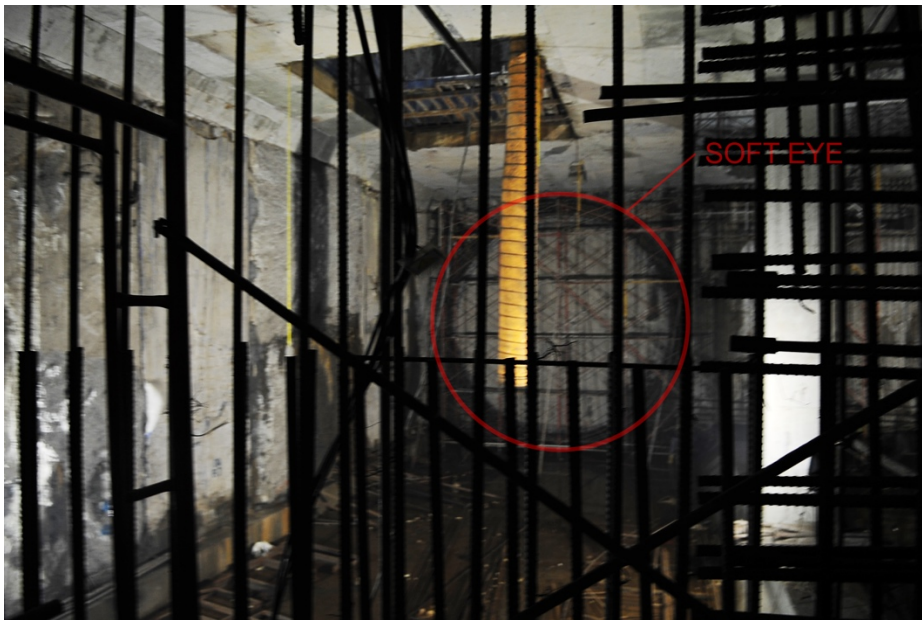
Figure 4.5: NSL-P2 tunnel soft-eye at the end of NSL-P1
