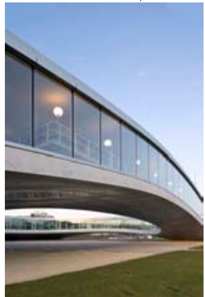
South Facade and view below towards Uni Lausanne photo: Ariel Huber
