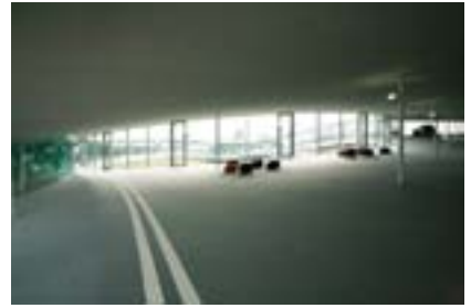
curved visually disabled guidance system photo: author
