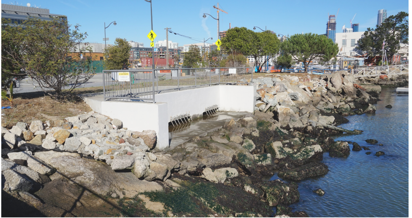
Figure 10.1: Rainwater discharge outlet in bay water, Source: (Author, 2018)
