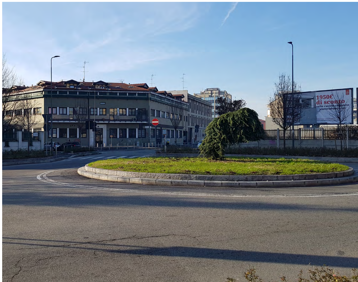
The second main roundabout offers a key big space for circulation and flow capacity management
