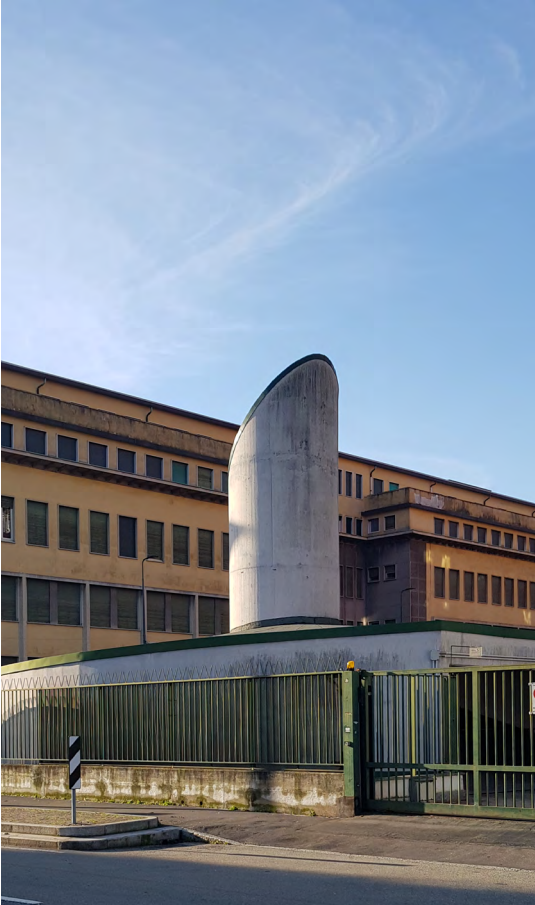
Signage flags exposed on the facade of the Event Centre
