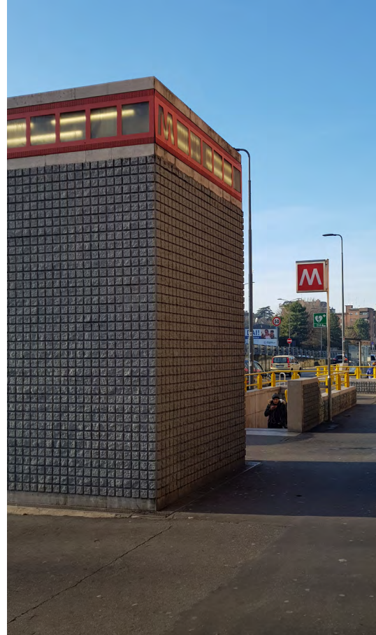
Lift access to the underground
