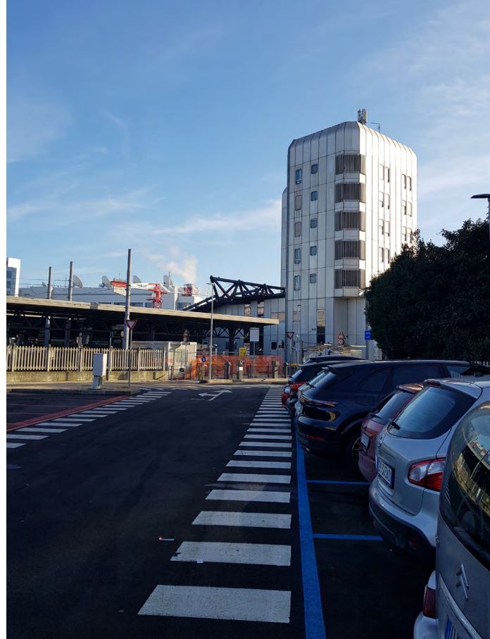
View of the Office tower from the carpark area
