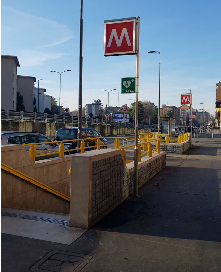
Pedestrian access to the underground
