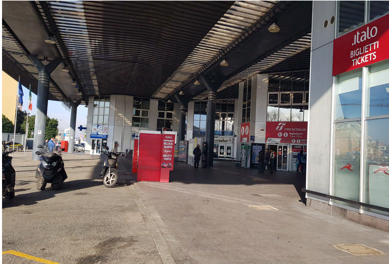
Rogoredo Train station main entrance High speed ticket office connecting Rogoredo to the rest of Italian's main cities: Venice-Bologna-Genova-Florence-Rome-Naples.
