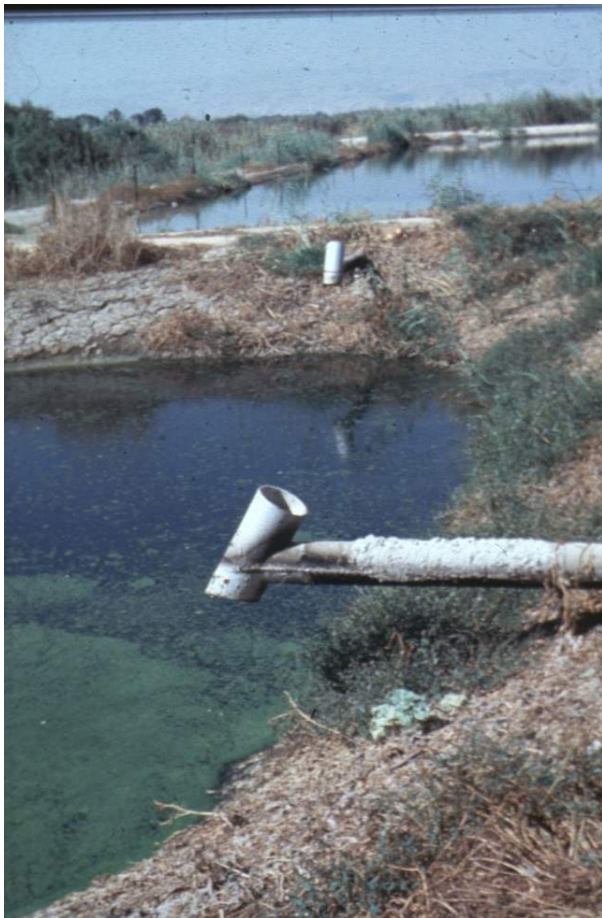
Figure 28: Image of a waste stabilization pond (van Lier & de Kreuk, 2014)
