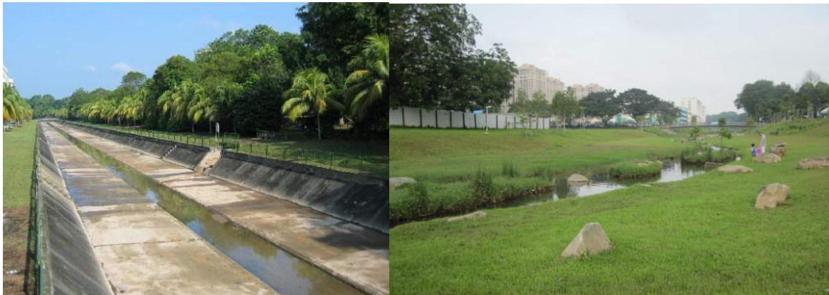
Figure 19: Restoring the riverbed of the Kallang River, Singapore. Pictures before (left) and after the restoration (right). (Chandrashekhara, 2015)
