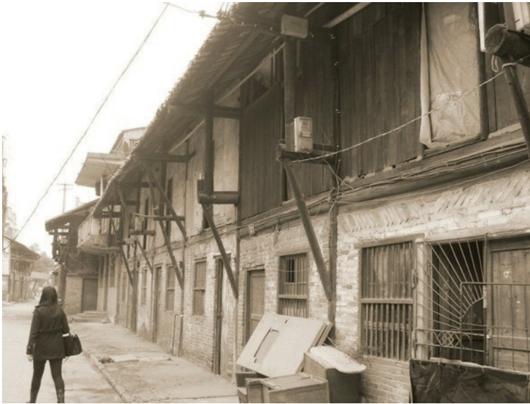
"beams over beams" to help reduce the number of the ground columns
