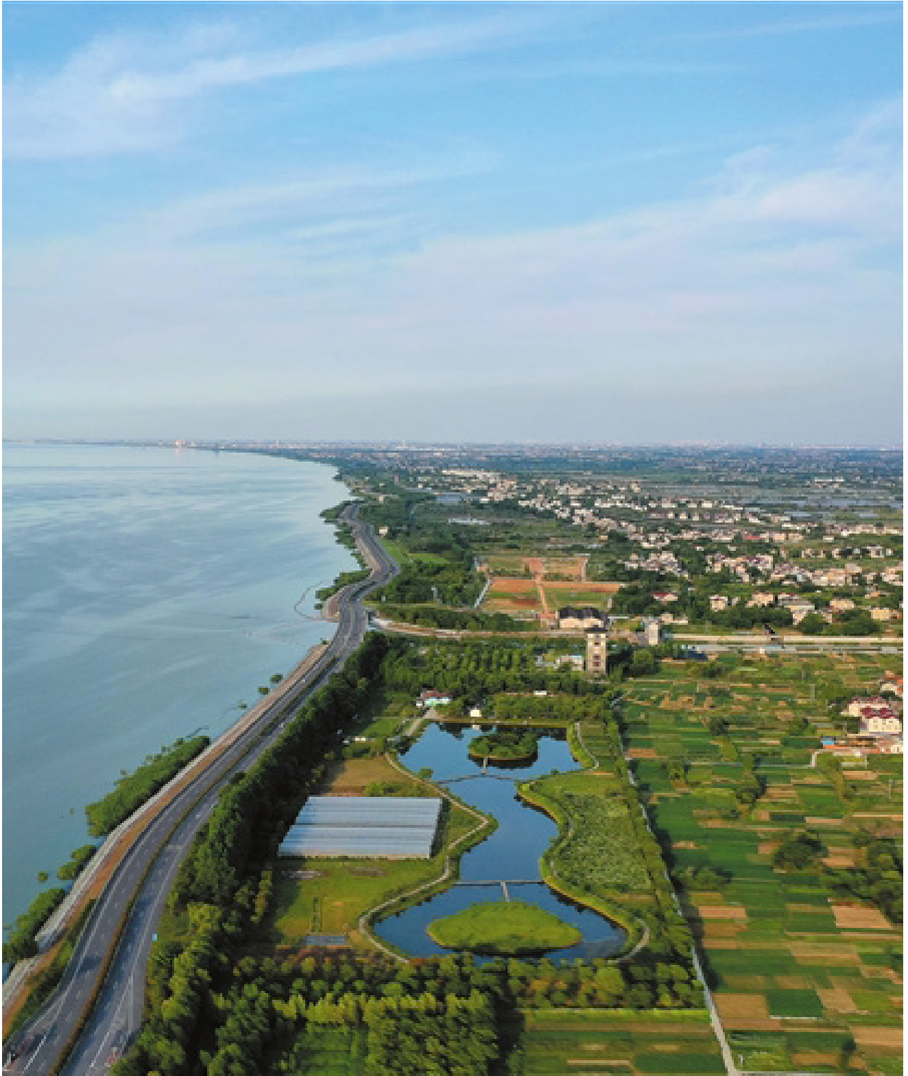
FIG. 178 Lougang polder in the Taihu Lake Basin
