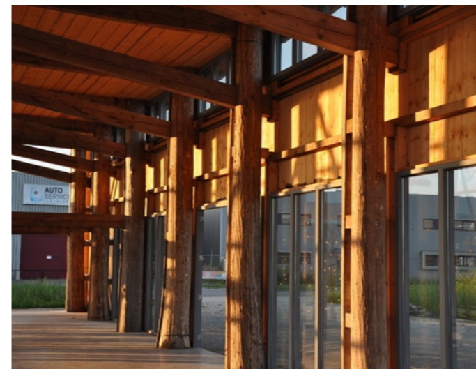
Figure 17: Construction workspace with poplar trunks as columns
