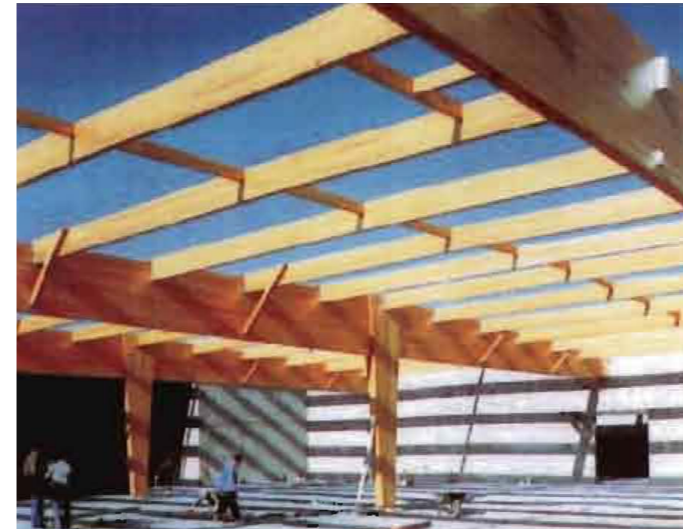
Figure 16: Construction with laminated poplar beams by Ets-Fournier
