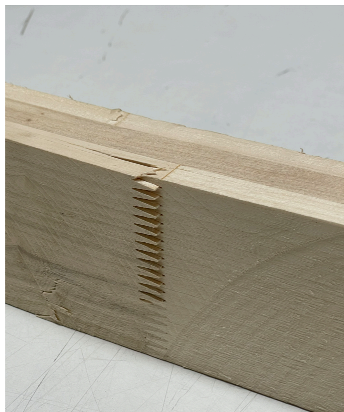
Figure 30: Failure of test piece 3 (L=398mm) at finger joint
