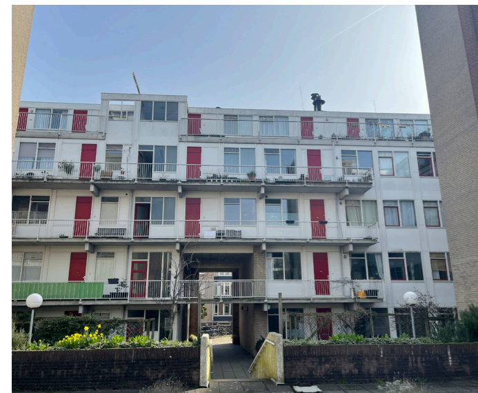
Figure 10: New façade of inner courtyard from 1987
