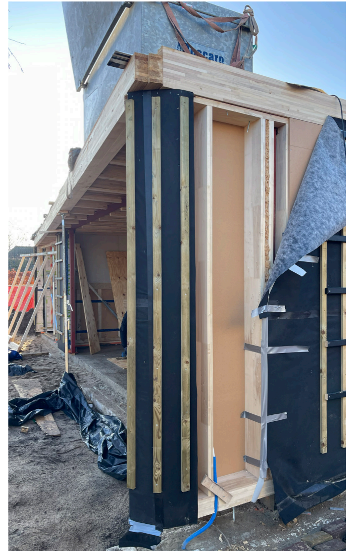
Figure 32: Assembly on site timber frame construction
