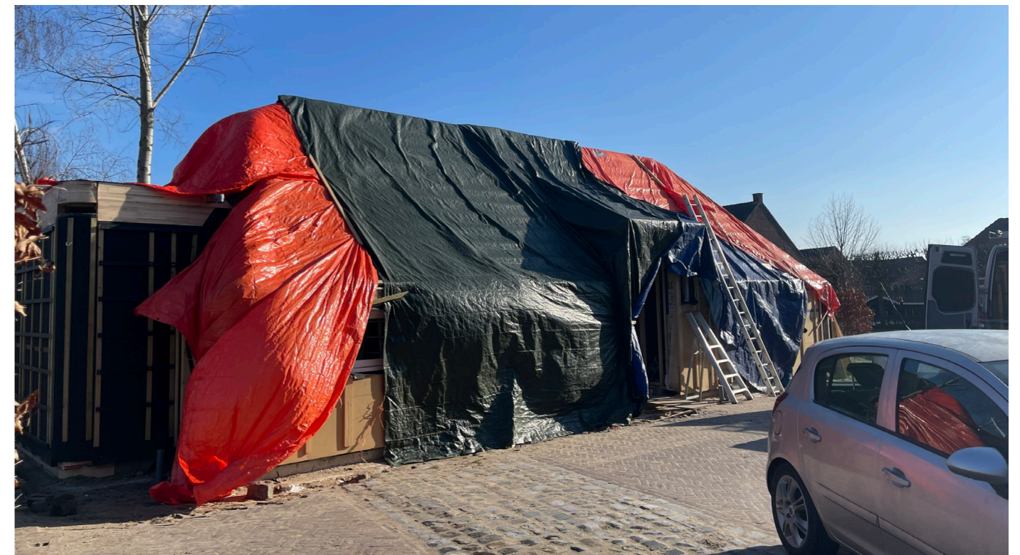
Figure 40: Covered construction site
