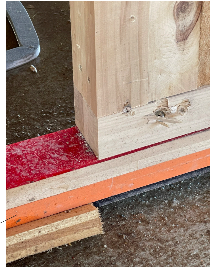
Figure 39: Connection poplar frames to concrete foundation
