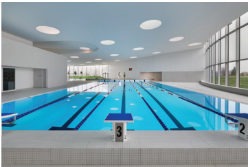
SWIMMING POOL COMPLEX
