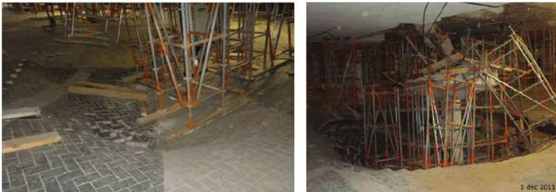
Figure 5.38, Deformation of the parking garage after failure. Source: Dossier Hageman 7998 sinkhole winkelcentrum 't Loon in Heerlen, 2012
