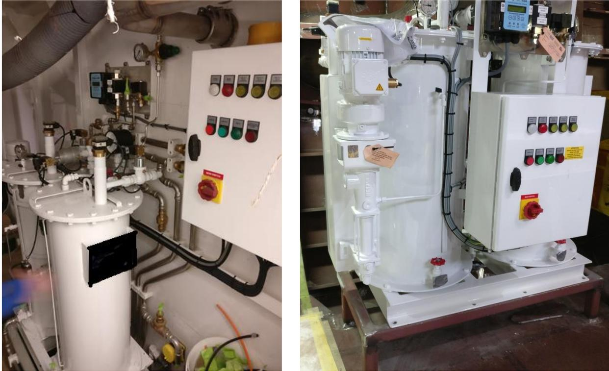
Figure 4-1 The complex version (left), and modular version (right)
