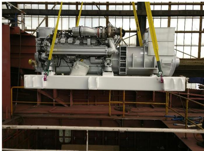
Figure 4-6 A generator is loaded in the engine room through the building hatch for the main engine
