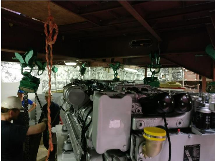
Figure 4-7 Manoeuvring a generator to its final position in the engine room
