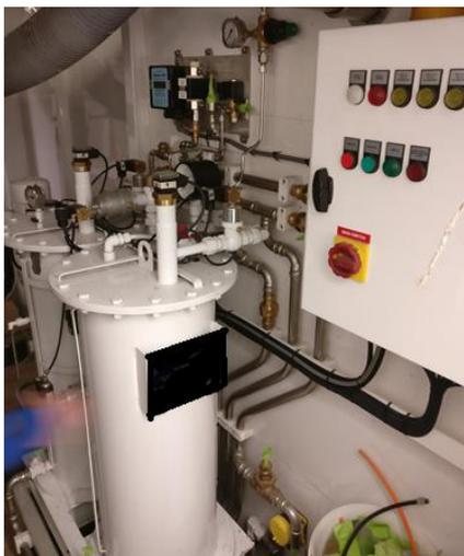
Figure 2 Complex oil-water separator
