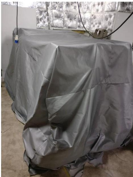
Figure 4-5 A generator protected by a welding blanket
