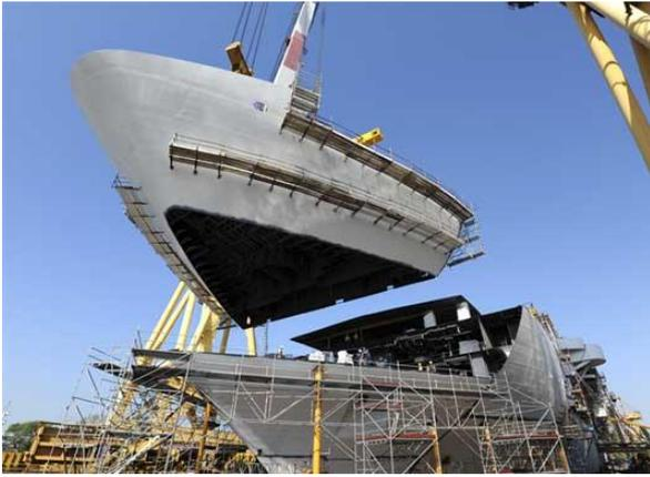
Figure 2-1 Block erection during the construction of a cruise ship
