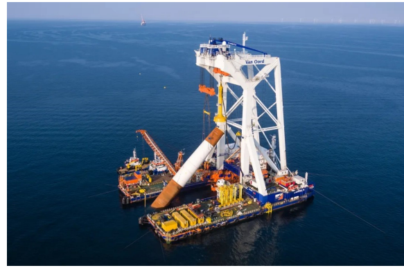
Figure 2.9: The heavy lift vessel Svanen performing a monopile upending operation [23].
