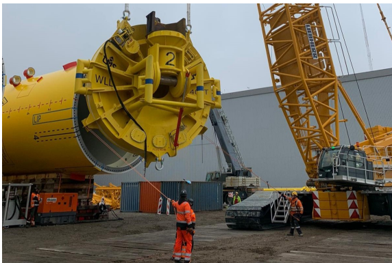
Figure 6.9: A pile plug being installed to make a monopile buoyant [85].
