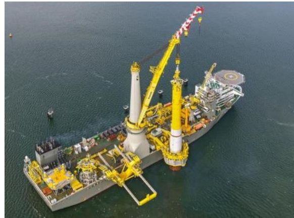
Figure 2.4: Monopile positioned within the gripper system alongside the installation vessel [13].
