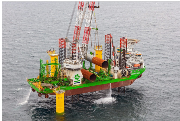
Figure 2.5: Purpose built Jack-Up Vessel DEME Innovation [16].
