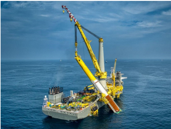
Figure 2.3: Monopile upending operation utilizing a deck-mounted upending hinge [12].
