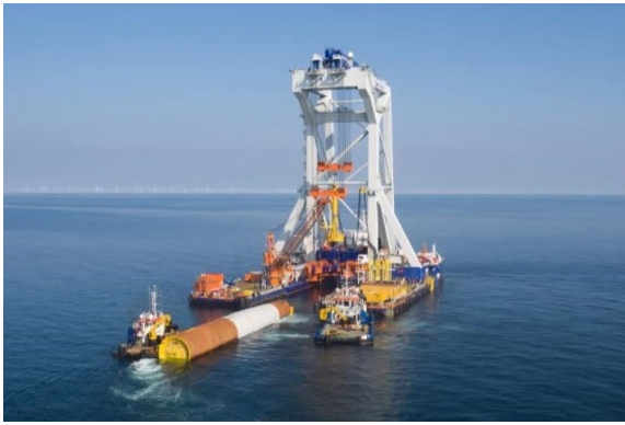
Figure 2.8: Floating monopile presented to Svanen by a tugboat [22].
