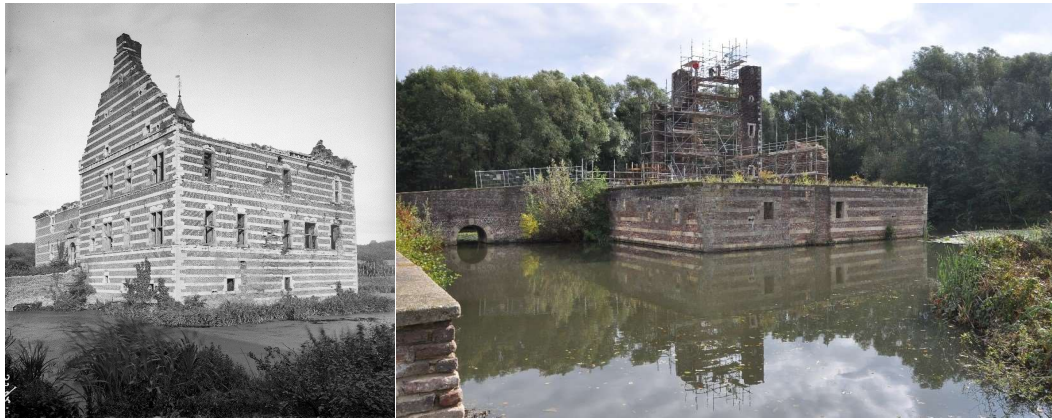
Figure 44- The castle in 1919, in comparison with the situation in 2014. Although the roofs and parts of the façades had been lost in the meantime, the castle was at that time in a considerably better condition than at the start of the recovery in 1975. (Photo: RCE) (Viersen, 2014)
