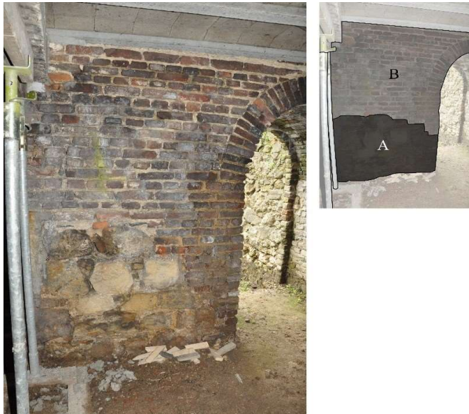
Figure 60- Overview of the tower cellar room, west wall, (Viersen, 2014)
