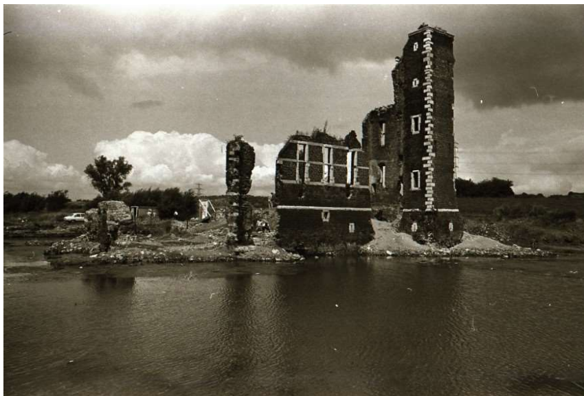
Figure 47- Overview of the ruin, seen from the south at the time of the excavation. The upper part of the narrow and high fragment on the left side of the still preserved part of the south façade is no longer present. (Photo: Hukkelhoven, Heemkundevereniging, (Viersen, 2014)
