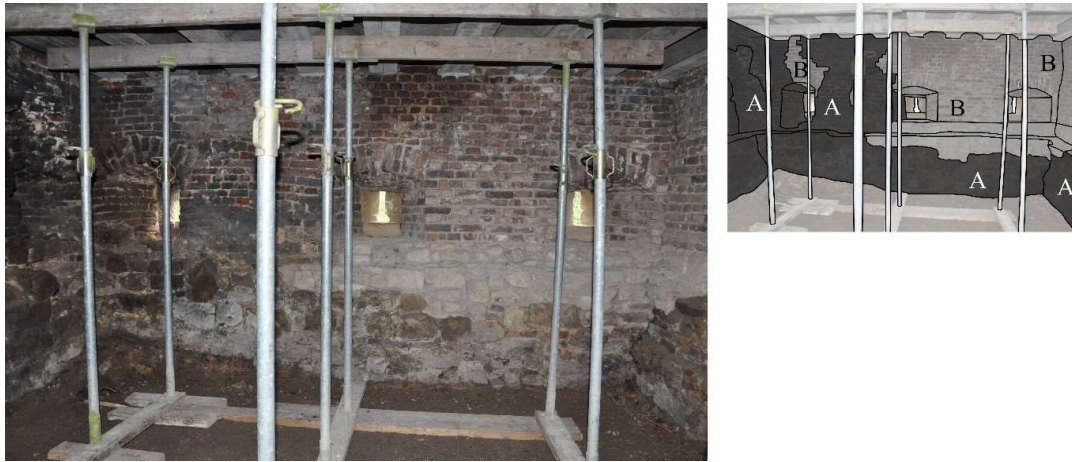
Figure 62- Overview of the tower cellar room, east wall, (Viersen, 2014)
