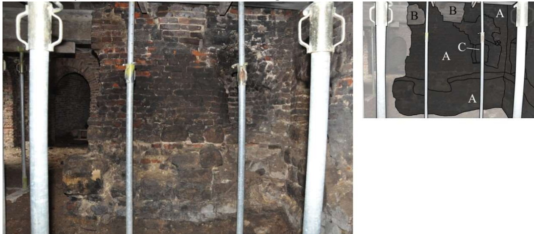
Figure 61- Overview of the tower cellar room, north wall, (Viersen, 2014)
