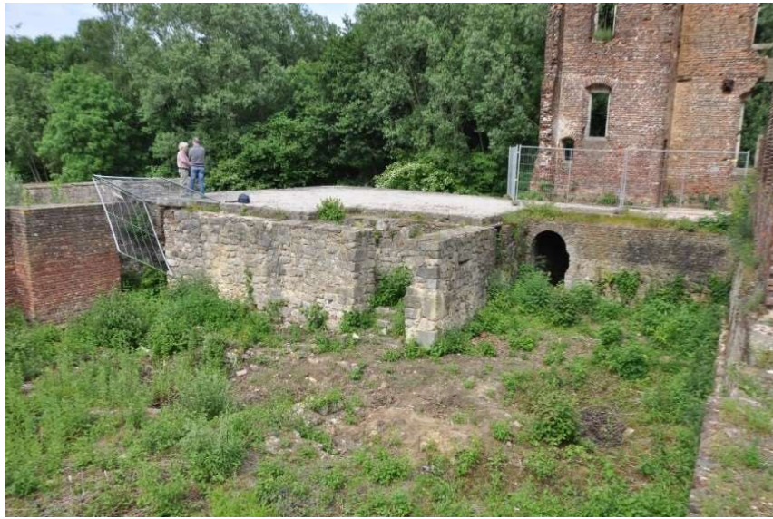
Figure 58- Overview of the largely reconstructed (rebuilt) brickwork that forms the walls of the former courtyard. Only on the underside of the walls there are some layers of the original masonry. The lower steps of the stairs are also original. (Viersen, 2014). See also the following image (Fig. 60).
