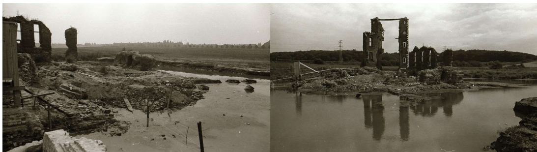
Figure 42- Overview of the castle at the start of the works in 1975. It can be seen that almost nothing remained above the canal level. The fragment of the west facade is the only part of the castle, of which something has been preserved above the water level. This means that
