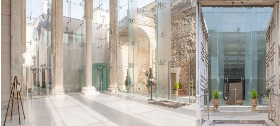
Figure 32- Restoration with glass of the ruins of the Augustan Temple in Pozzuoli (Naples Italy), Gnosis Architettura and Bardeschi 2011, retrieved from divisare.com
