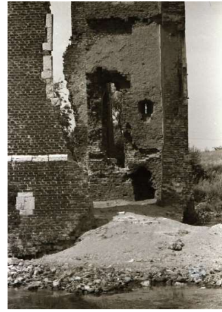
Figure 50- Left: the castle, seen from the southwest. The west facade of the tower is almost entirely original. Right: the south facade of the tower before it was consolidated. Shortly before taking this photo, the southeast corner of the tower collapsed. The basement is still partly filled with debris. On the outside, the masonry was heavily damaged by watering. The masonry of the outer wall has probably been lost below the water level. On the inside, the brickwork has been preserved up to about a meter above the level of the basement. If the canal had not been dug out in the 1950s, the corner of the tower would probably not have collapsed. (Photo: Hukkelhoven, Heemkundevereniging, (Viersen, 2014))
