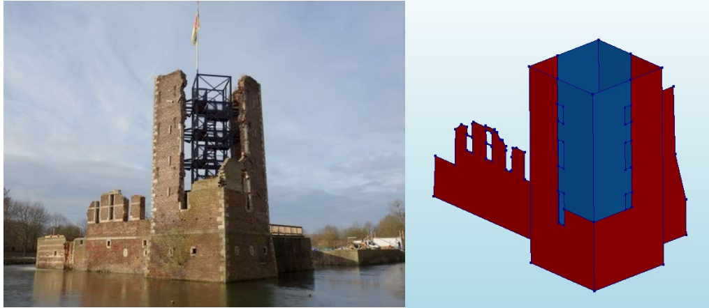
Figure 85- Overview of the Castle Ruin with the present steel staircase consolidation
