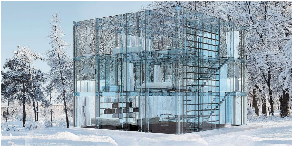
Figure 18- The glass house Santambrogiomilano, 2010, Milan, Italy retrieved from https://www.santambrogiomilano.com/the-glass-house
