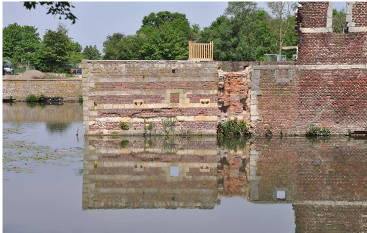
Figure 48- Overview of the castle south façade, western part, (Viersen, 2014)
