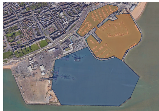
Figure 5.2: Zoomed satellite image of Ramsgate, with the port area (blue) and marine area (orange) shown. (Google Earth, 2024)
