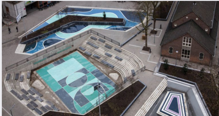
Water Square Rotterdam, De Urbanisten
