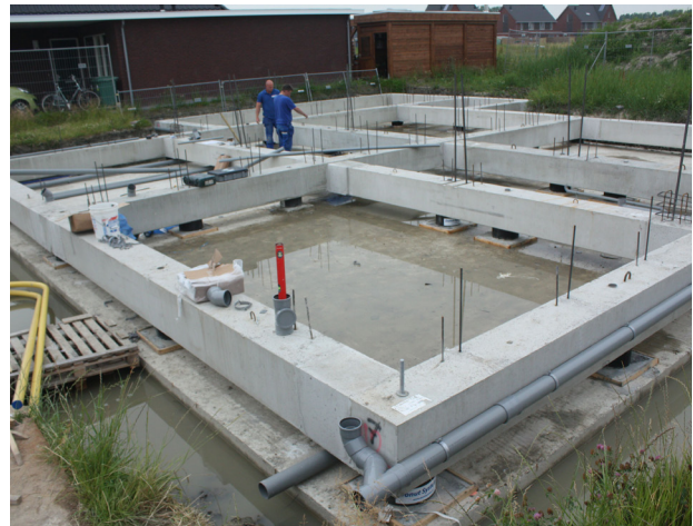
Figure.59: DONUT-system base isolation | Source: Plegt-Vos
