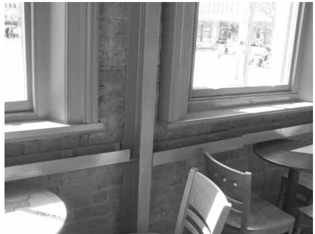
Figure.49: Steel strongbacks in the interior | Source: Dizhur
