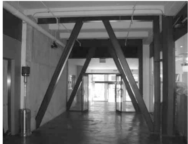
Figure.53: Addition of a steel frame | Source: Dunning Thornton consultants:
