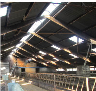
Figure.23: Interior of barn with timber frames in Loppersum | own image
