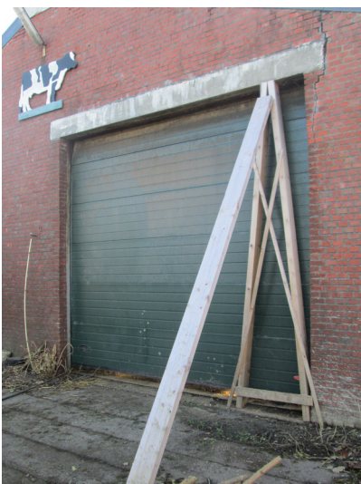
Figure.21: Entrance of a barn shed in Loppersum | own image
