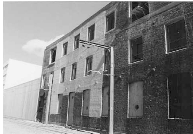
Figure.51: FRP applied to a wall | Source: Dunning Thornton consultants
