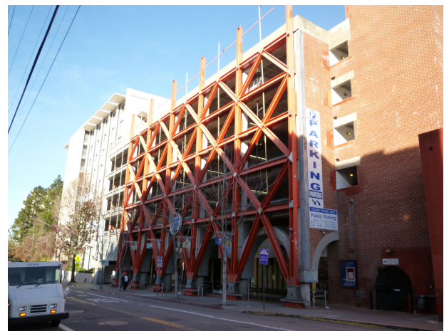
Figure.74: External placing of seismic resisting elements
