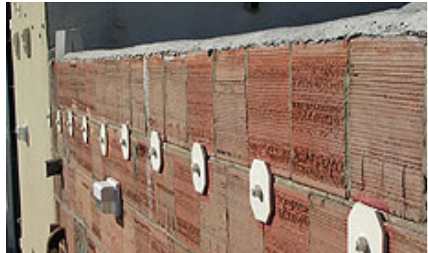
Figure.45: Added wall-diaphragm anchors | Source: San Diego government
