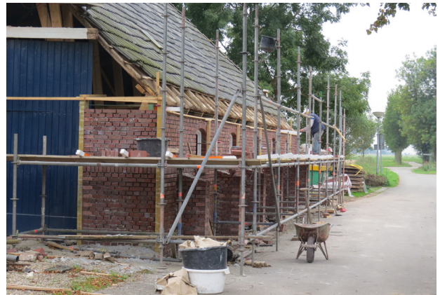
Figure.2: Site visit: renewal of farm wall, Loppersum | Own image
