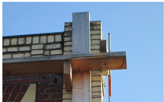
Figure.42: Temporary tensile tying of the facade, Loppersum | Own image
