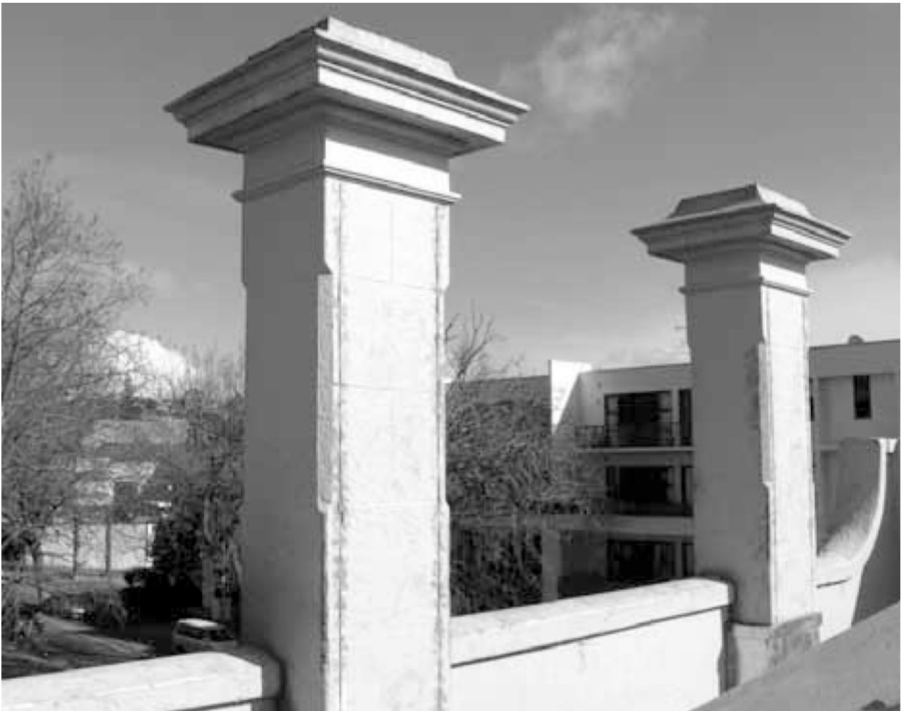
Figure.39: Parapet strengthening with near-mounted FRP strips | Source: : Dizhur
