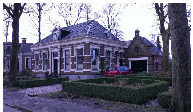
Figure.72: House at stationsstraat in Loppersum. Adapted to assess the building respectively with chimney, with FRP chimney and without chimneys
