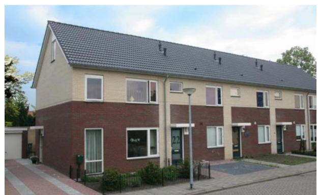
Figure.66: Masonry buildings in the Netherlands | Source: Wijte (2014)
