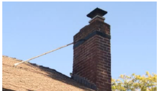
Figure.4.4: Chimney braced towards the roof | Source: KGW
