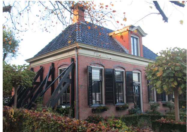
Figure.40: Temporary timber shoring, Loppersum | Own image
