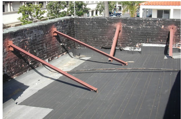
Figure.4.3: Parapet bracing | Source: Structural Renovations
