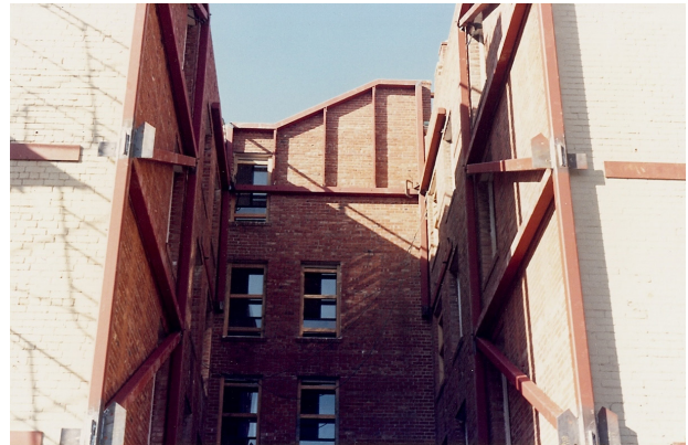
Figure.73: External placing of seismic resisting elements
