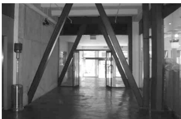
Figure.70: Intrusive steel braced frame in a hallway | Source: Dunning Thornton consultants
