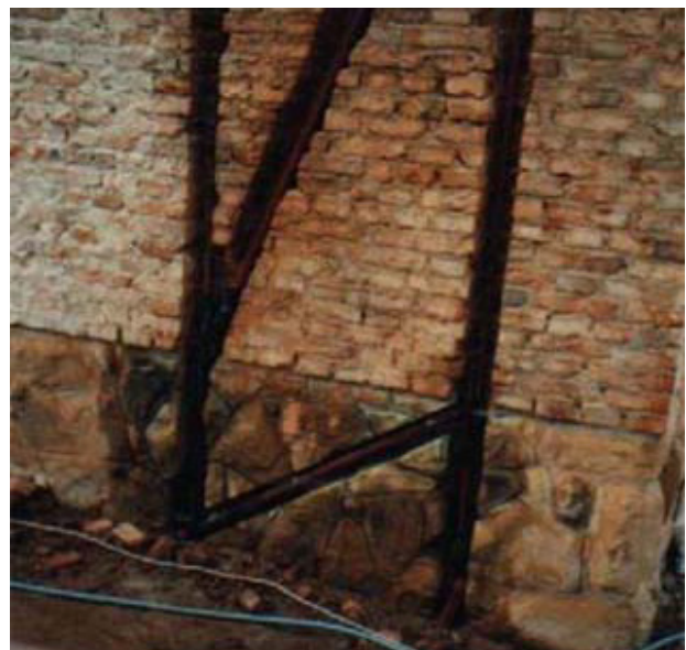
Figure.58: Implementation of dampers into brick wall apartment houses Source: DC 90
