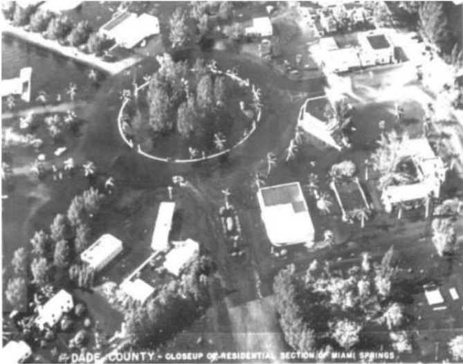
Flood in Miami Springs 1950s
