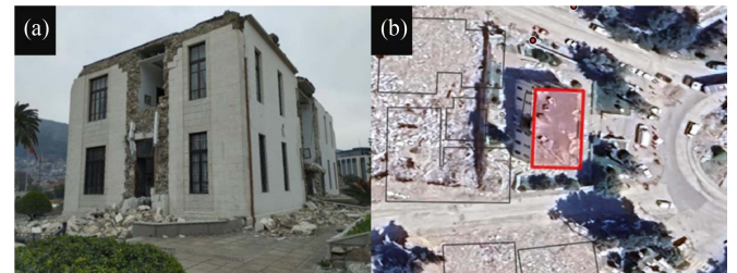
Fig. 11. Building with a damage grade of 4 on the EMS-98 scale in Antakya with damaged sides. Panel A is a photograph from the 13–17 March 2024 survey. Panel B is a MAXAR image on 8 February 2024 of the same building, with building footprints from the Microsoft dataset [26]. The footprint of the building is displayed in red. Despite being classified as “very heavy damage” in the field survey, the AI-based damage assessment computed the damage as 0%.
