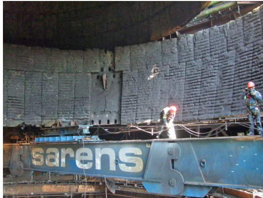
(b) More sophisticated heavy lift beam with couplings
