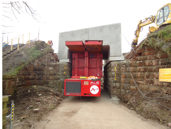
Figure 2.9: Application where a vertical spacer is required [3]
