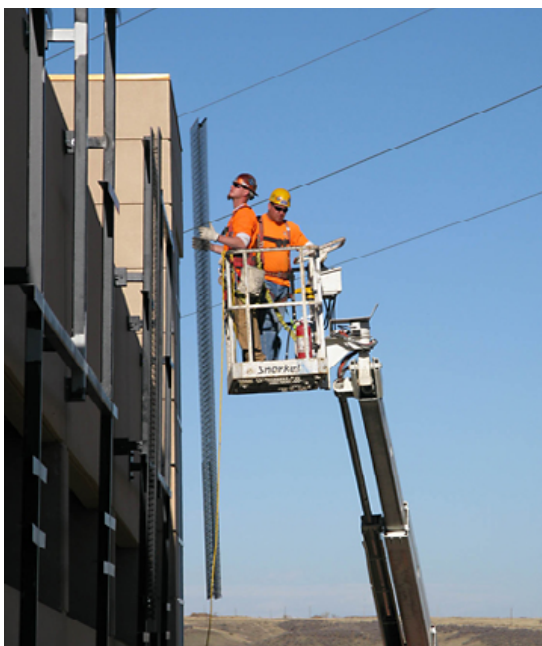
Installing panel system façade greening: source: Greenscreen p.7
