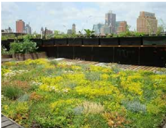
sedum mixture semi-extensive green roof
