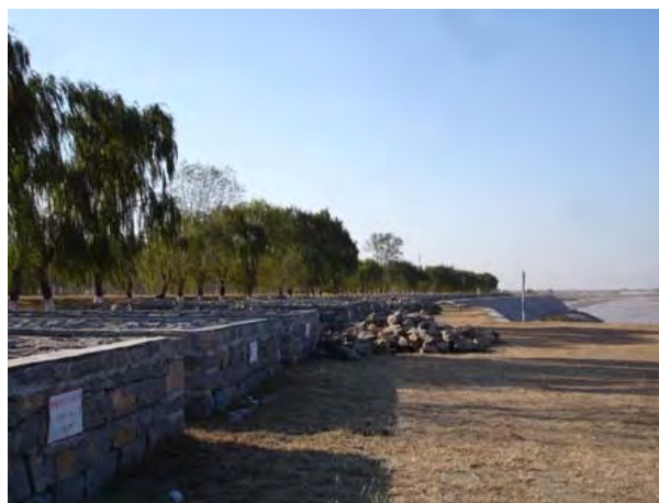
Well-laid rock on dangerous section
