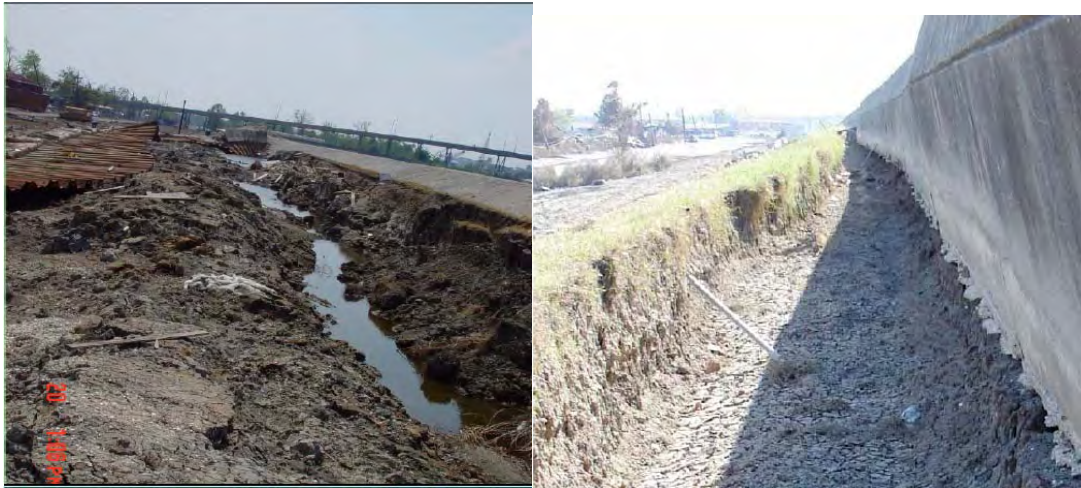
Figure 3.18 Example of breach along IHNC (east side) from overtopping and scour (top) and scour behind adjacent section that did not fail (bottom)
