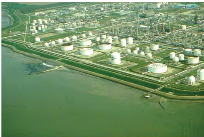
Figure 4.15 Refiners on artificial mound in Rotterdam (Source: Rijkswaterstaat)
