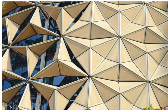
FIG. 1.18 Responsive façade of the Al Bahr towers in Abu Dhabi by Aedas architects. From 'Flickr' by © Inhabitat, 2014 ( https://www.flickr.com/photos/inhabitat/12330988375/sizes/l/ ). Licensed under CC BY-NC-ND 2.0
