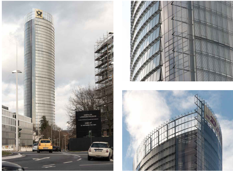
FIG. 4.16 Post tower in Bonn by Murphy & Jahn architects
