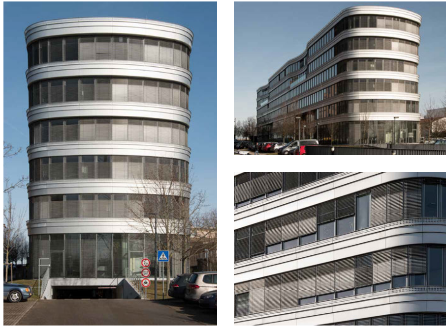
FIG. 4.12 Z_Zwo in Stuttgart by Eike Becker architects
