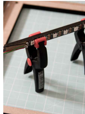
FIG. APP.D.10 Installation of LED strips to visualize the heating and cooling function
