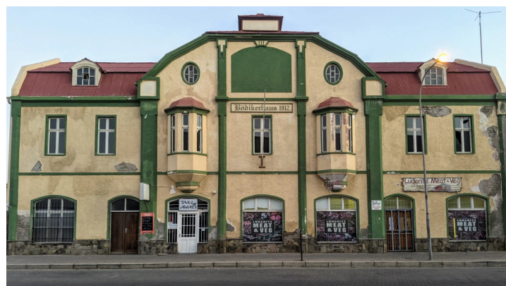
Figure 13.16: Front view of the Bodikenhaus
