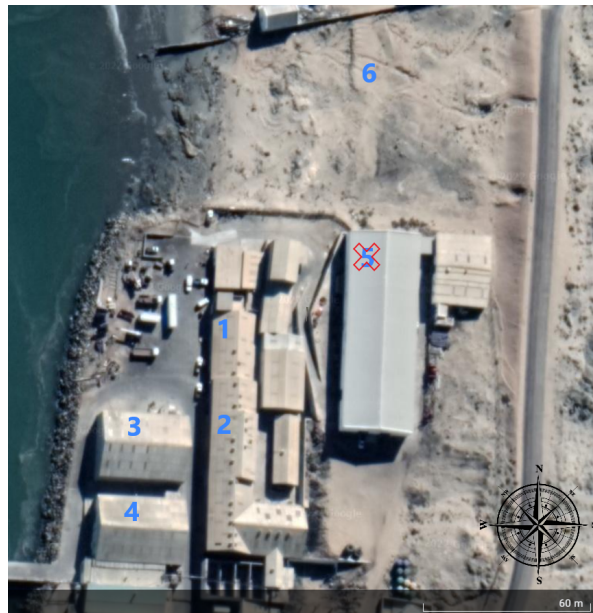
Figure 13.18: Overview different buildings of Lalandii workshop
