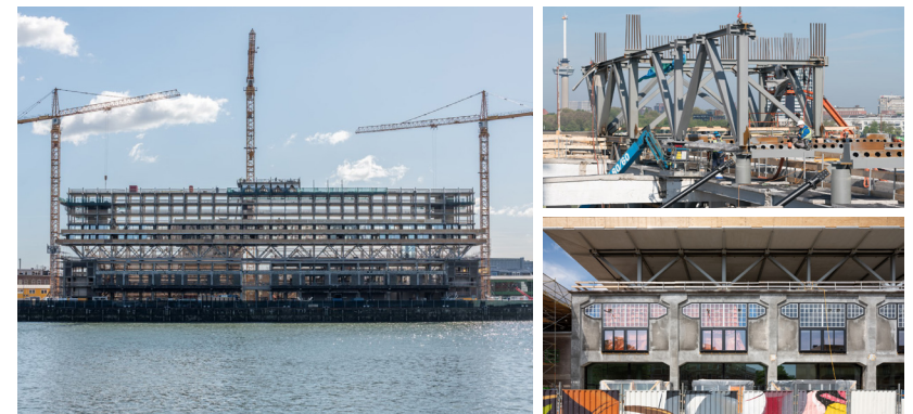
Figure 110. A) The dwellings have a smaller grid size than the hall below B) The transfer layer bridges the difference in grid sizes (Mei, 2019).
