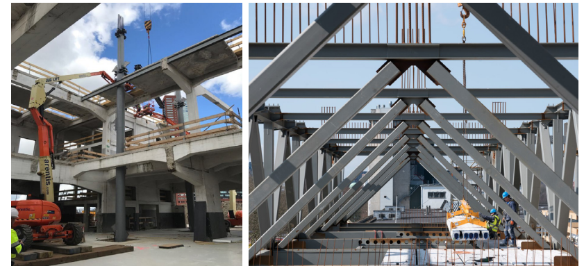
Figure 109. A) Careful positioning of the new structural columns. B) the transferstructure allows for minimal perforations (Mei, 2019).
