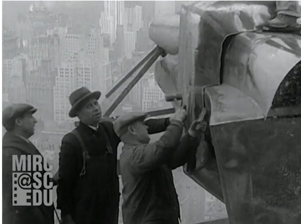
Figure 20: Scene from a construction footage of the Chrysler Building. In this image workers were hammering an eagle ornament into a suitable shape to mount it.
