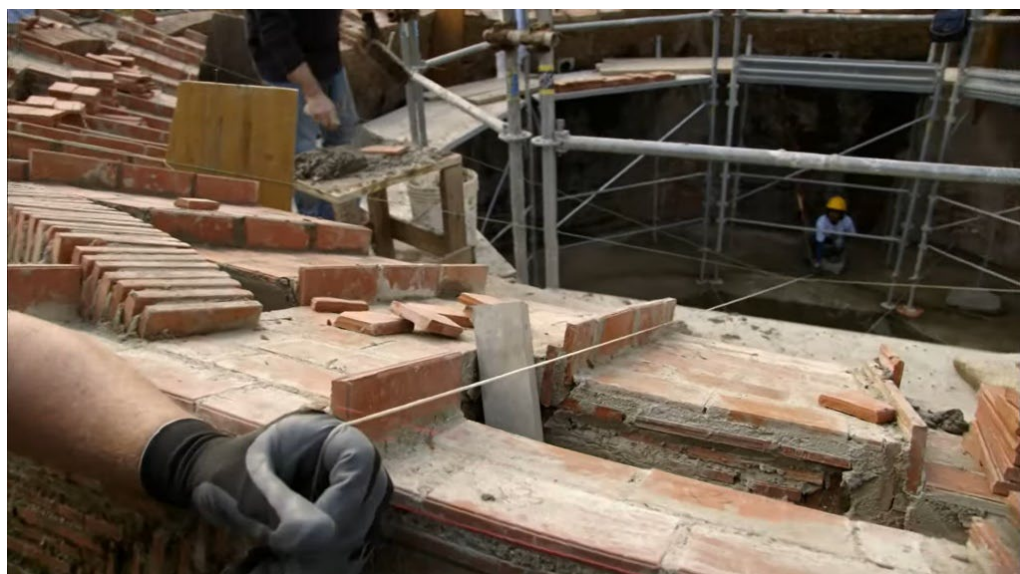
Figure 17: Top: 1:5 dome reproduced by team led by Massimo Ricci. It demonstrated the self-supporting capacity during construction.
