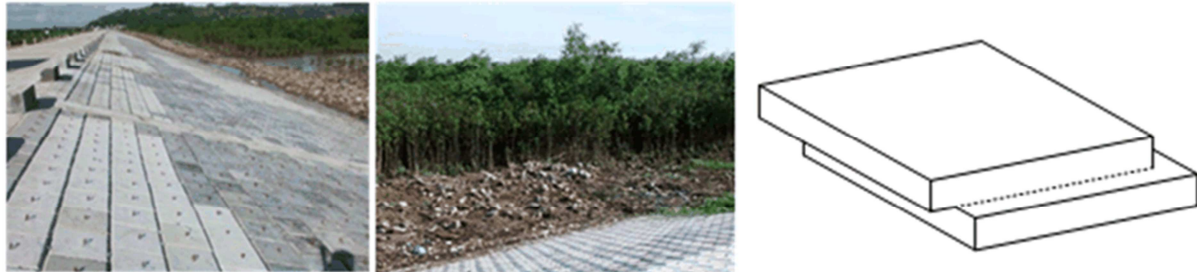
Figure 2-14 Sea dike #2 in Do Son with concrete block 40x40x24 cm
