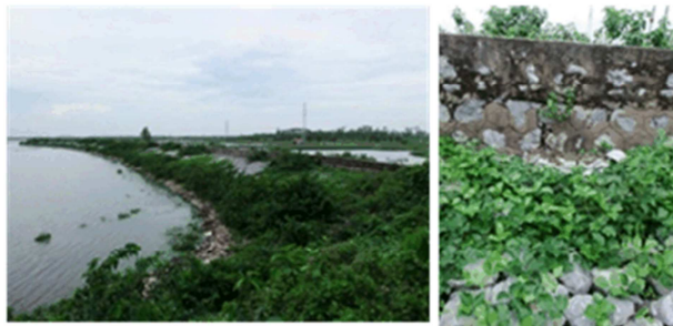
Figure 2-18 Sea dike of Tinh Quang Ninh with rip-rap revetment
