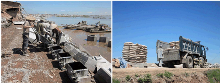
Figure 2-34 Filling the formworks and the supply of raw materials
