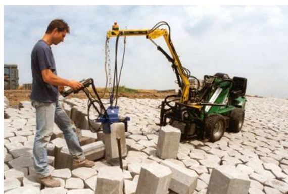
Figure 9-2 Placing by hand with small machine
