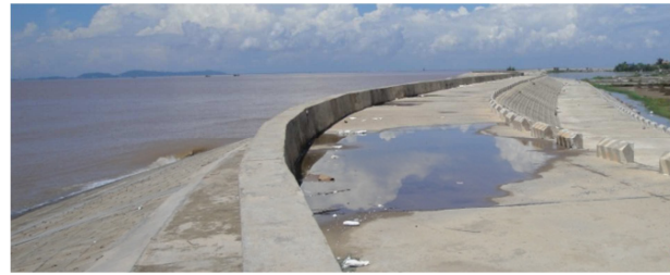
Figure 5-1 Sea dike at Cat Hai Island.
