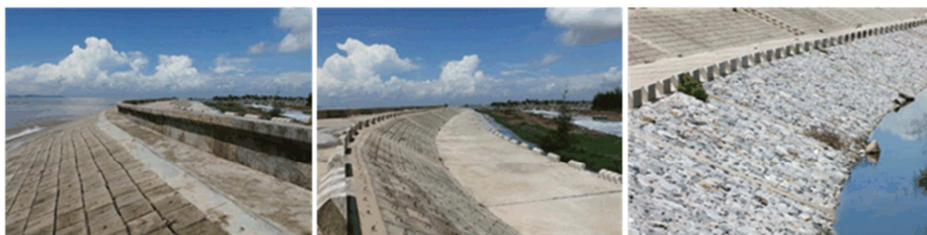
Figure 2-8 Test dike #2 on Cat Hai Island with flat concrete blocks
