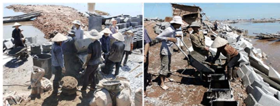
Figure 2-32 Mixing concrete and putting it into the formworks
