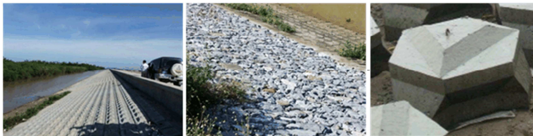
Figure 2-12 Sea dike #1 in Do Son
