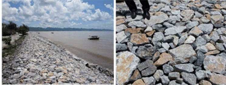
Figure 2-10 Rip-rap revetment dike on Cat Hai Island
