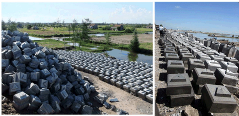
Figure 2-35 Storing and curing blocks on site
