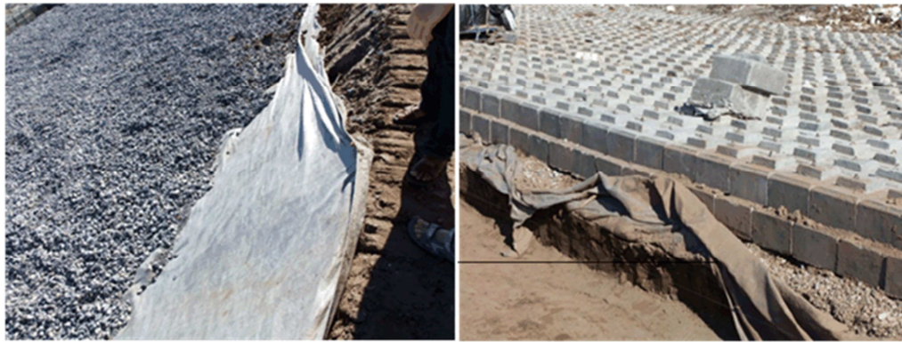
Figure 2-38 Placement of stone layer and geotextile
