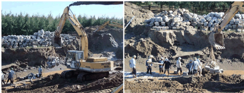
Figure 2-36 First part placing by crane
