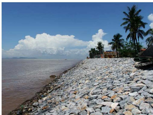
Figure 2-22 Rip rap dike
