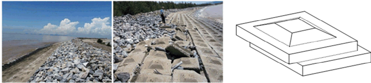
Figure 2-5 Test dike #1 on Cat Hai Island with concrete interlocking blocks 60x60x28 cm
