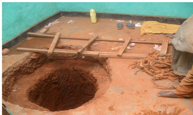
Fig. 3. Pit latrine being created inside the room of a house in Biryogo settlement.
