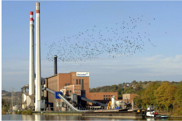
Figure 2-1: Les Awirs power plant
