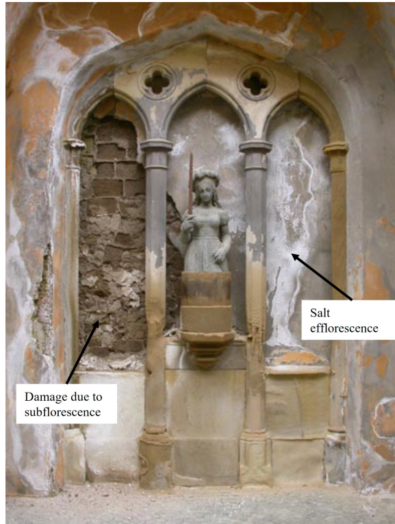
Figure 2.1: Example of salt damage to a lime-based render, garden wall of Stolzenfels Castle [3]. The left panel shows spalling of the render caused due to subflorescence (in-pore salt crystallisation). The right panel shows presence of salt efflorescence (minor aesthetic issue)
