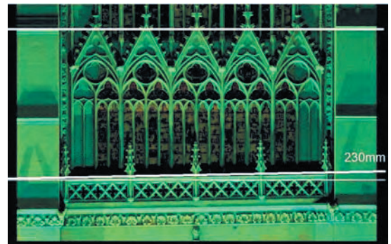
▲ Figure 6: Misalignment of the balcony of the south facade of Notre-Dame Cathedral in Amiens.
