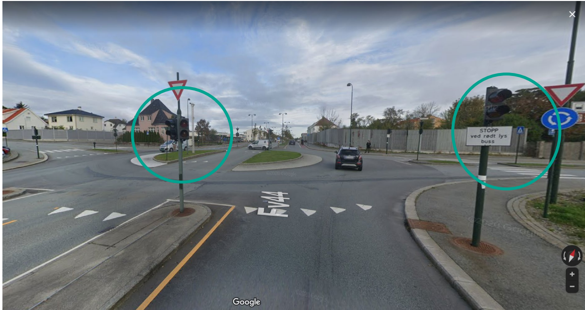
Figure 13 Roundabout on Hillevågsveien in Stavanger, Norway. Picture from google maps street view.
