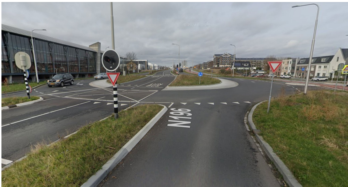
Figure 11 Picture of a throughabout on N196 in Aalsmeer, Netherlands. Picture from Google Maps Street view.
