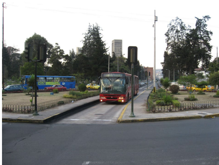
Figure 6 BRT solution with an exclusive lane through the centre island of a roundabout (ITDP, 2017)
