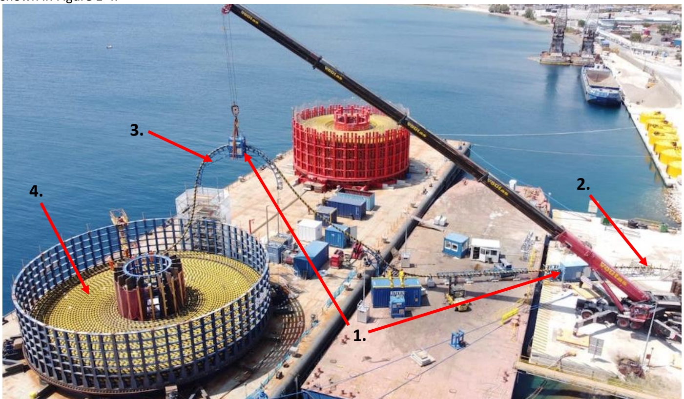
Figure 1-4: General cable carousel (un)spooling setup [6]
