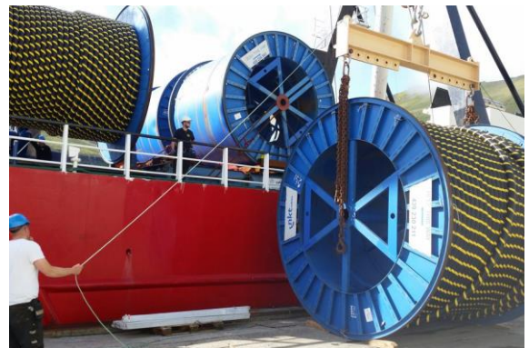
Figure 1-7: Transportation offshore power cables with reels [9]
