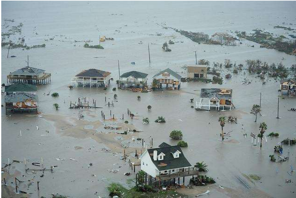
Figure 3 Damage caused by Hurricane Ike (Harper, 2015)
