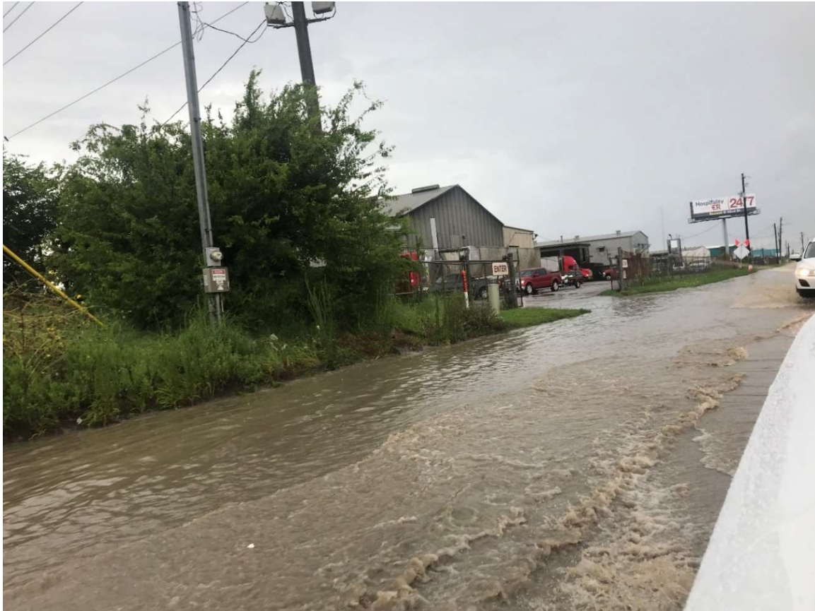
Figure 146 Flooding on Harborside Dr (Photo courtesy of authors)
