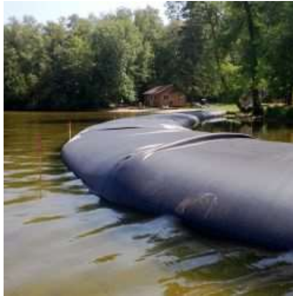
Figure 60 Example of a floatable barrier (Dam-It Dams, 2018)
