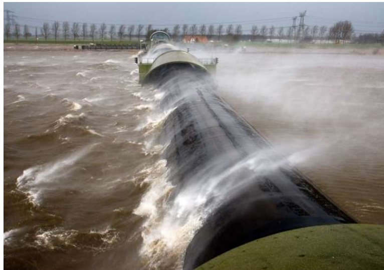
Figure 59 Ramspol barrier in the Netherlands (Rijkswaterstaat, 2017)
