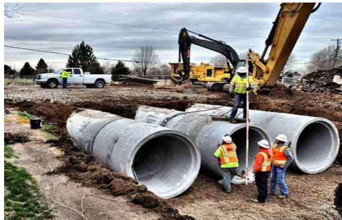
Figure 78 Installation of concrete drainage pipes (American Concrete Pipe Association, 2018)
