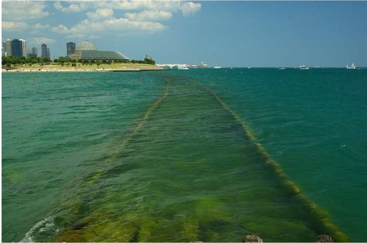
Figure 50 Submerged breakwater (Lech H Photography, 2012)
