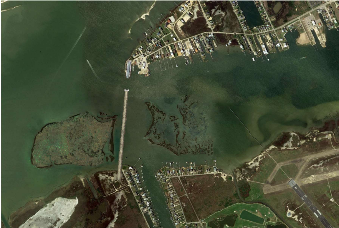
Figure 63 Offatts Bayou ecological barrier in open configuration
