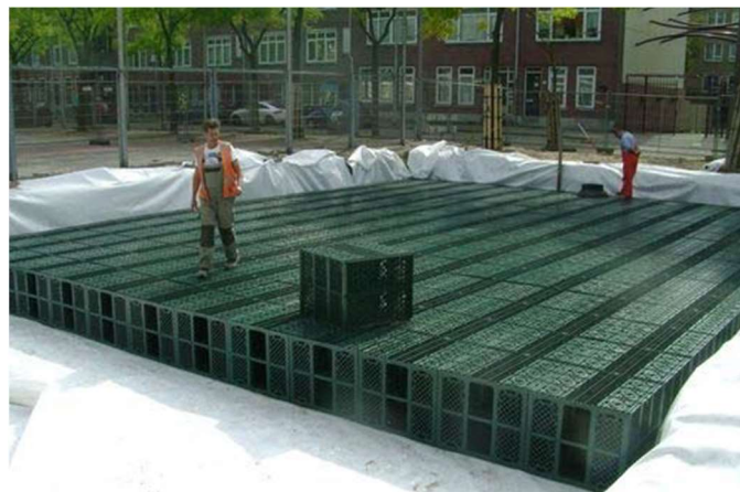
Figure 80 Installation of infiltration crates (WaterWindow, N.D.)
