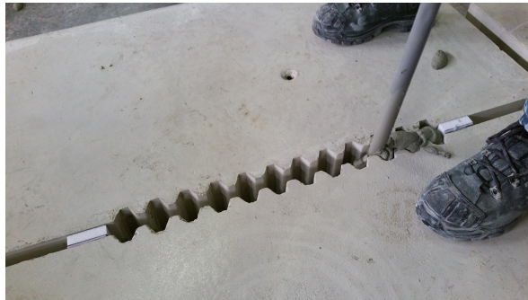
Figure 4.10: Inserting the mortar with a hose
