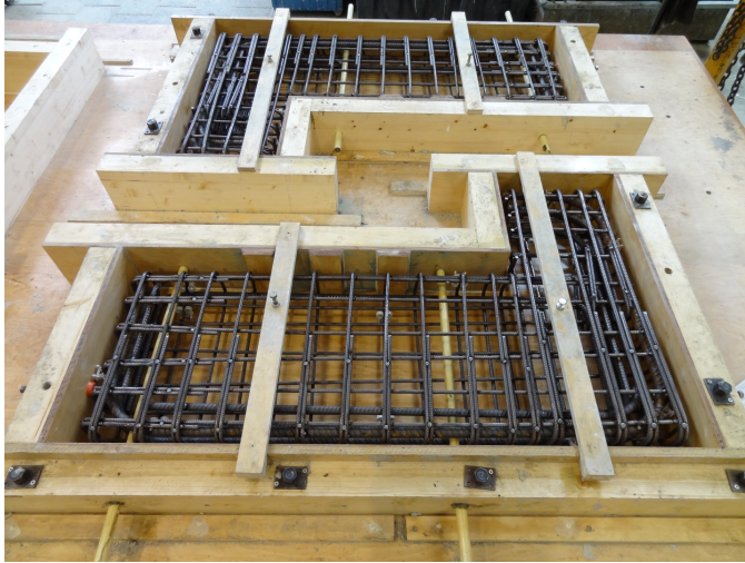
Figure 4.6: Construction of L-elements in the concrete factory
