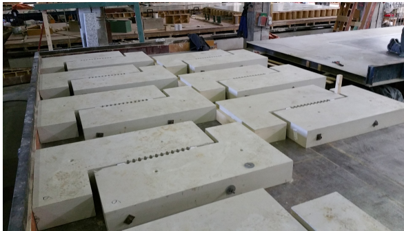
Figure 4.8: Construction of specimens in the concrete factory of Bestcon
