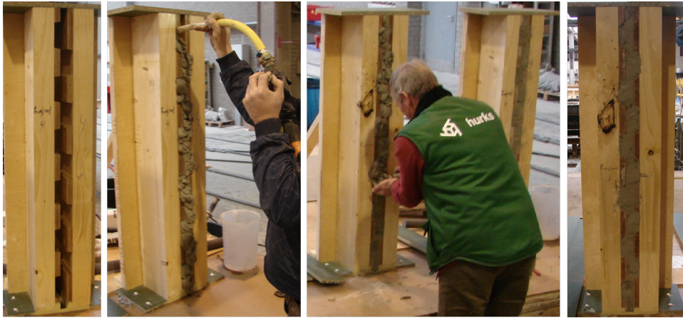
Figure 4.2: Testing the filling of vertical seams with mortar pump
