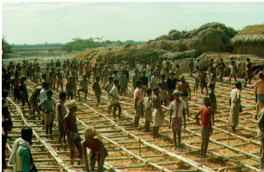
Figure 13-9 Construction of bamboo mattress
