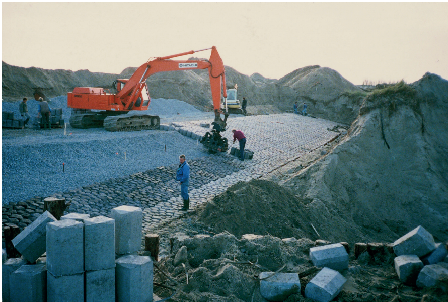
Figure 13-21 Mechanical placement of Basalton (RWS, Hans Johanson)
