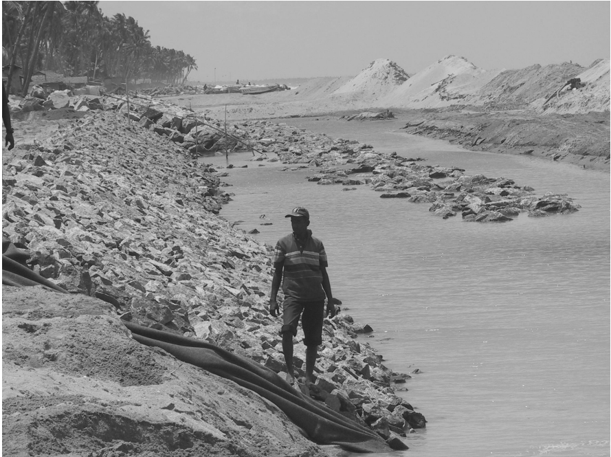
Erosion protection in Sri Lanka (photo Pilarczyk)
