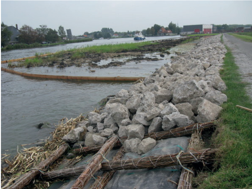
Figure 11-8 Geotextile under mattress (photo Griendhouhandel)
