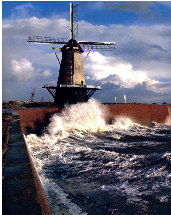
Figure 11-27 Seawall (Vlissingen, photo Wil Riemers)
