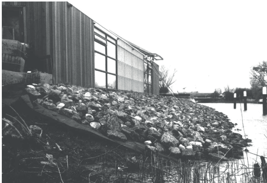
Figure 11-16 Simple bank protection with geotextile
