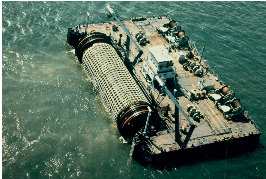
Figure 13-10 Sinking block mat in Eastern Scheldt (Rijkswaterstaat)
