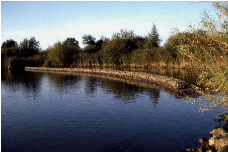
Figure 12-21 Wave reductor
