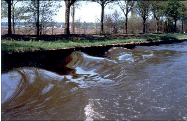
Figure 11-18 Sheet pile wall along canal (photo CUR)
