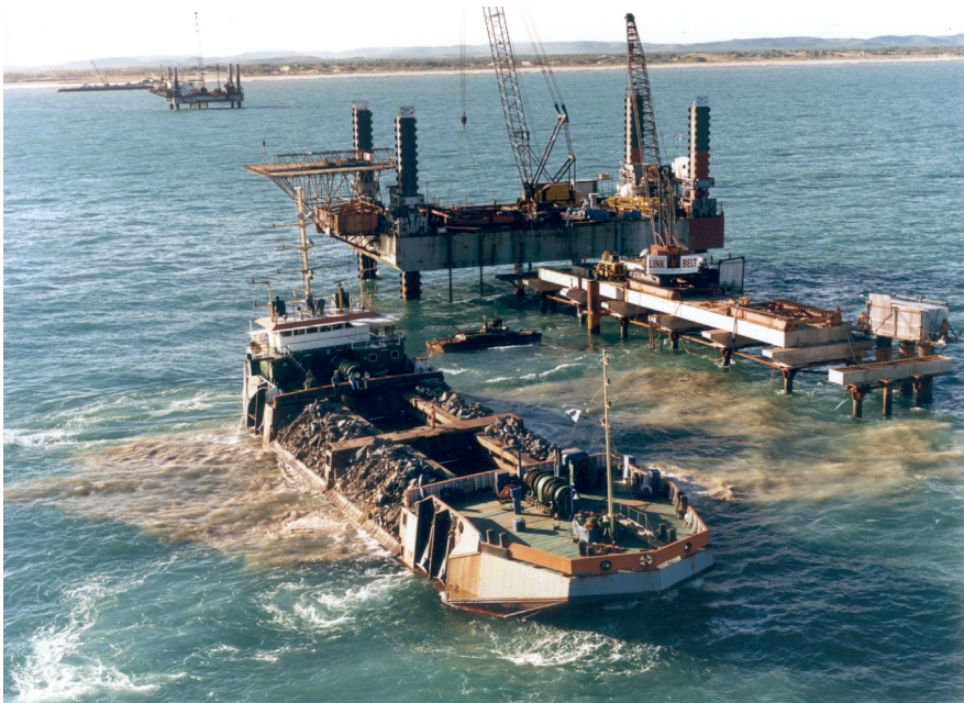
Figure 13-5 Side stone dumping vessel (Boskalis)
