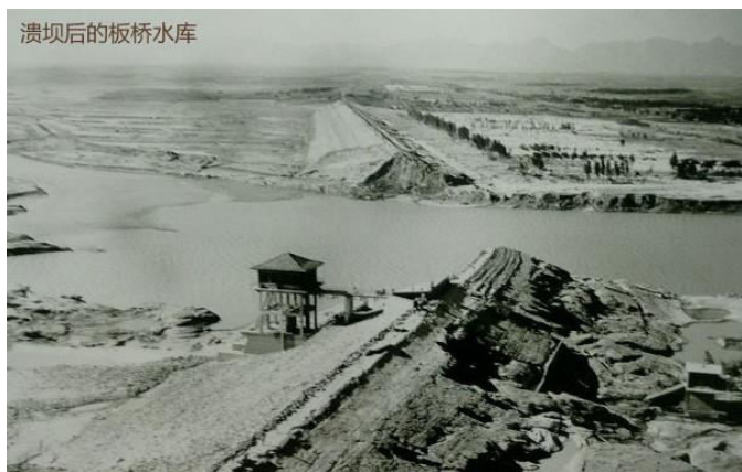
Figure 2 The breached Banqiao dam in 1975.
