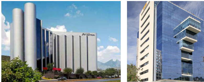
Fig. 8 Examples of round (left) and rectangular (right) shape façade of the sample
