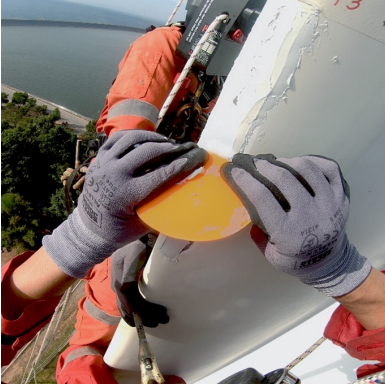
(a) Rope technicians applying a leading-edge repair product; photograph reproduced from Belzona (2022).
