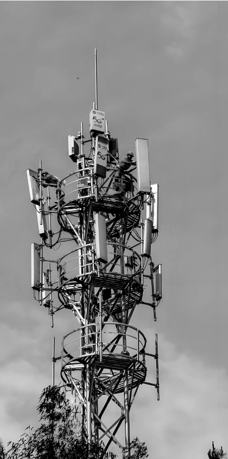
Fig. 3.16, Cell Tower Cell towers provide wireless connectivity between users' devices and the broader cloud network.
