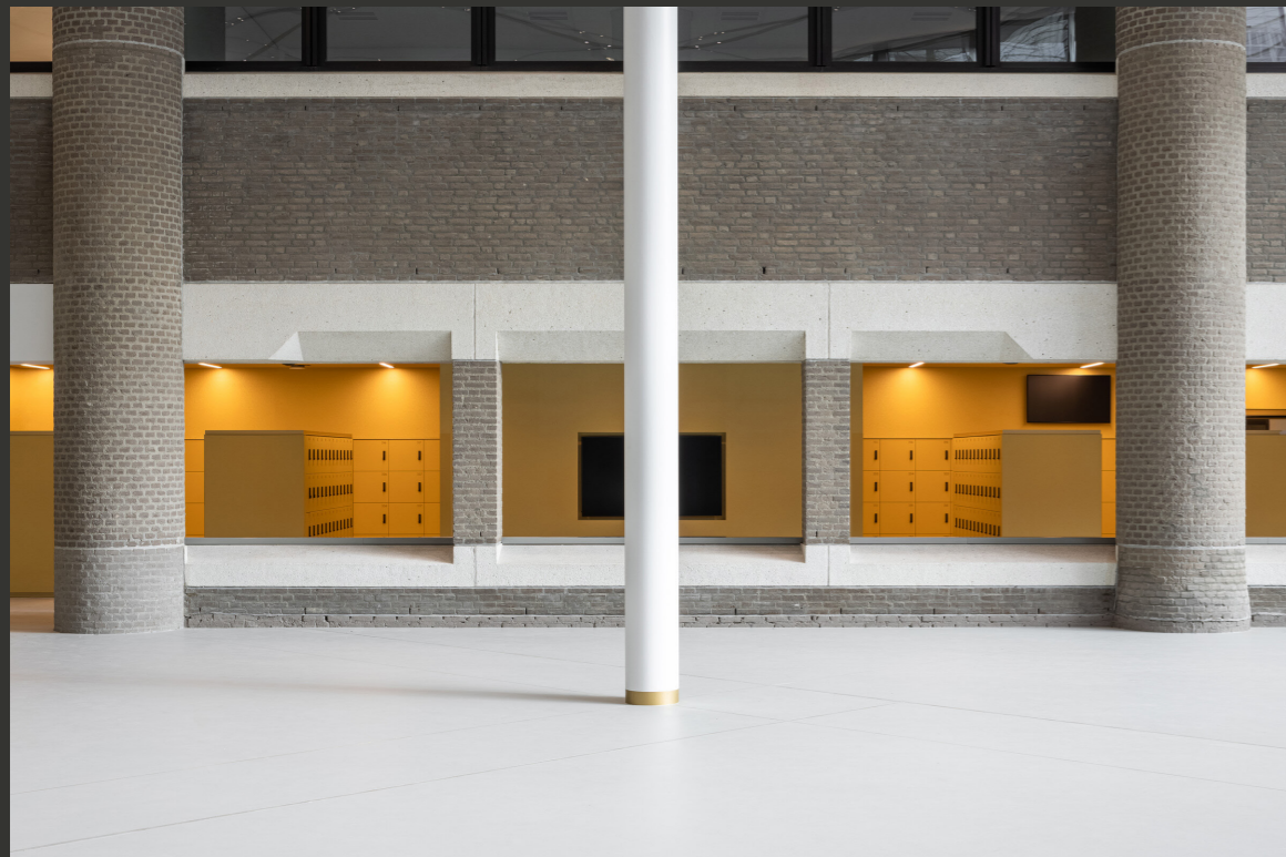
Figure 48 / Old and new construction. Poelstra, 2021.
