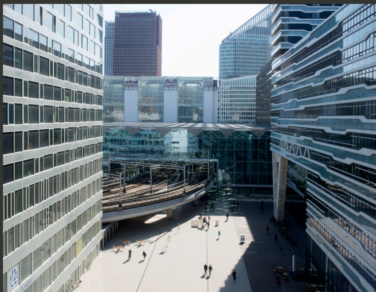
Figure 37 / The square next to Den Haag CS, the building of University of Leiden and New Babylon. Ministerie van Buitenlandse Zaken, 2014
