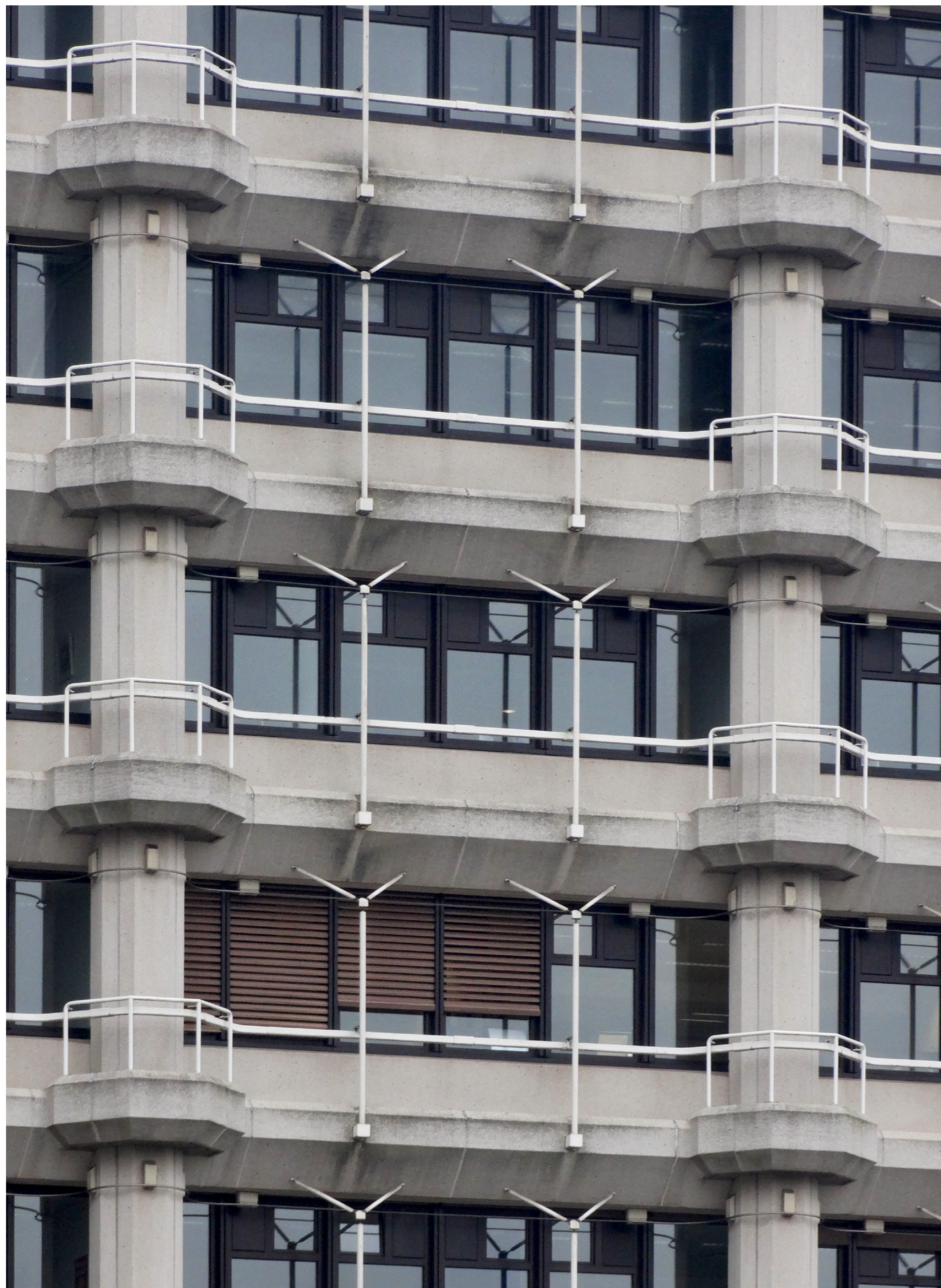
Figure 43 / Facade, upper part. Own image, 2024.
