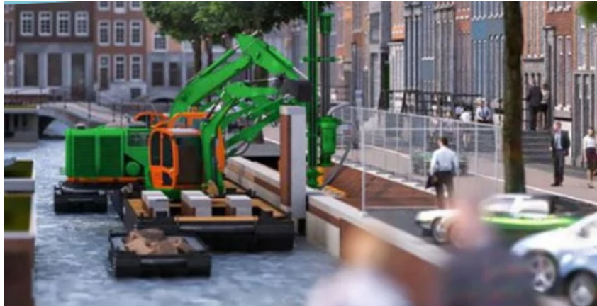
Figure 3.2: The work in Koningsgracht is done from pontoons. [4]
