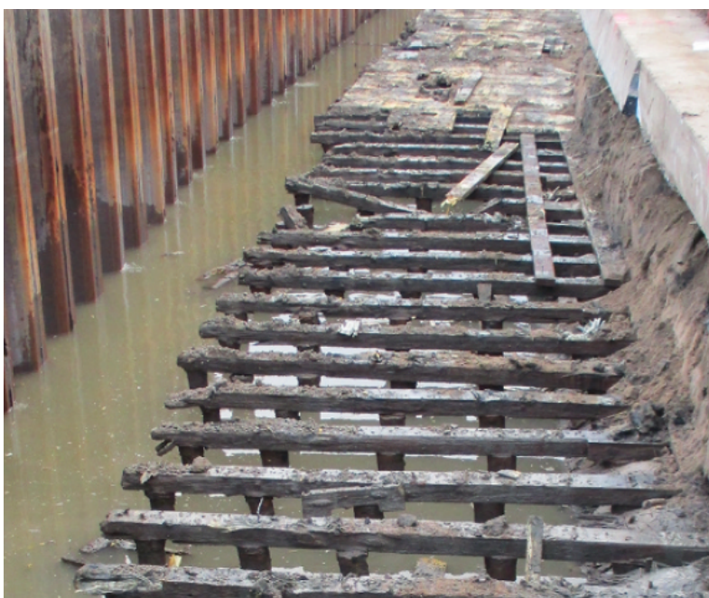
Figure 4.2: The exposed timber cross beams of the Maaskade in Rotterdam. [22]
