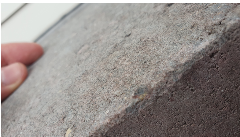
Figure 7.4: The smooth surface of the concrete bricks.
