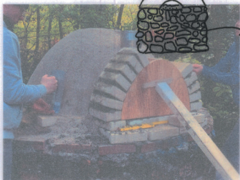
Making the dome out of sand
