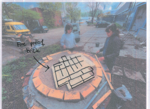
Making the top layer of the base with steel-framed concrete/clay and finishing it with fire-proof bricks
