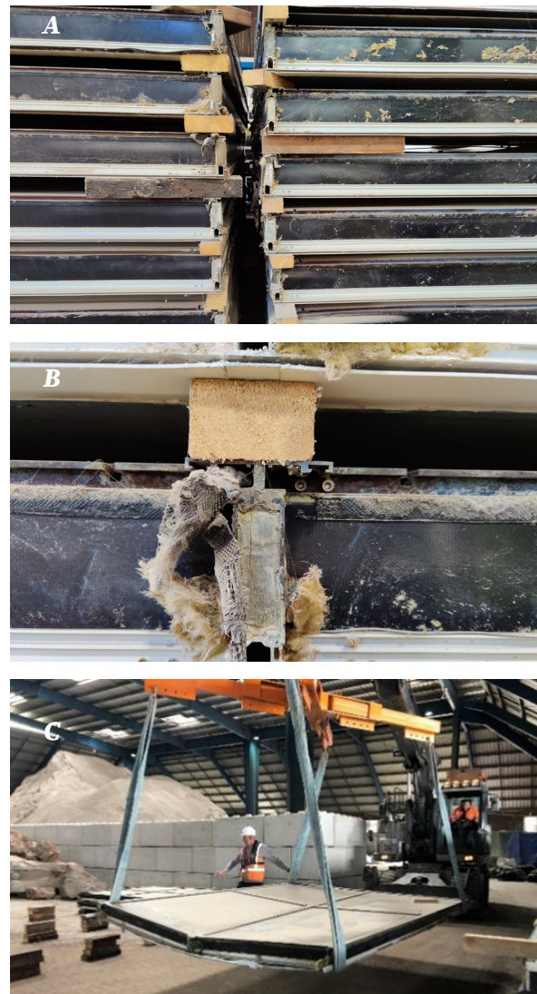
Figure 71 - A & B: The present condition of the units in the storage facility near Amsterdam. C: Shows the way the elements were transported. Source: Author (Pictures A & B), captured during a site visit. & Alkondor (Picture C)
