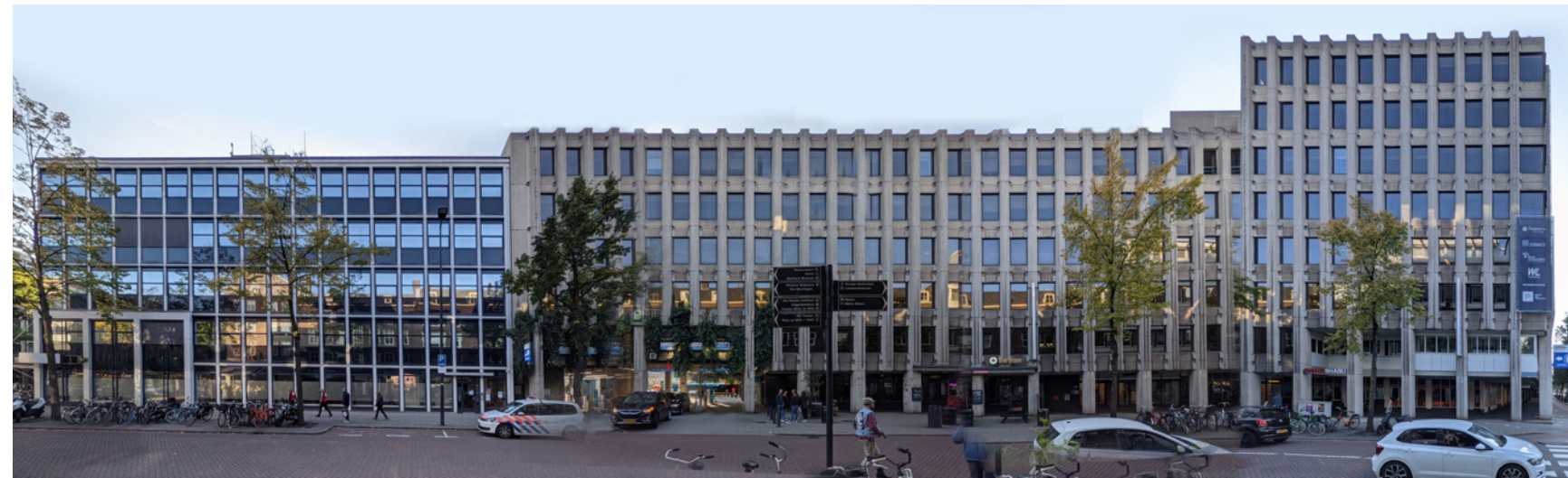
Figure: Hartmansstraat elevation and the former police station on the left end
