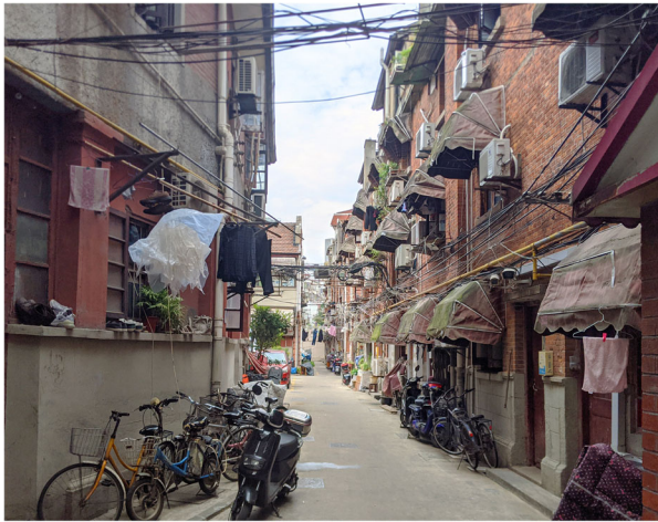
Fig. 5 The organized terraced buildings in Bugaoli, constructed with red bricks and timber window frames and door panels on the architectural façades (Source: Kaiyi Zhu, 2018)
