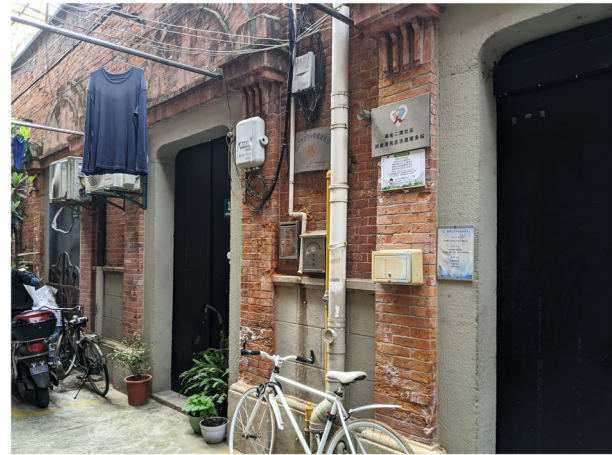
Fig. 7 There are newly added elements on the façades, such as equipment for fire safety and the white sewage outlets (Source: Kaiyi Zhu, 2018)
