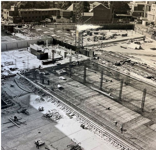
Concrete reinforcement
