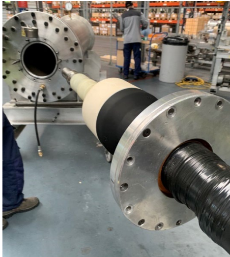
Figure 6.19: Prepared stress cone and cable prior to installation in the chamber
